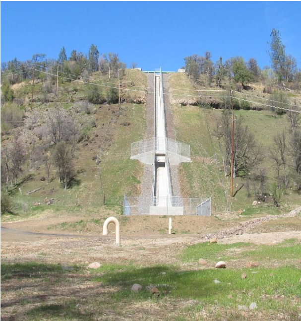
Before (left photo, January 2011) and after (right photo, March 2013) construction, uphill view of the new Inskip Powerhouse penstock bypass at the chute section.
