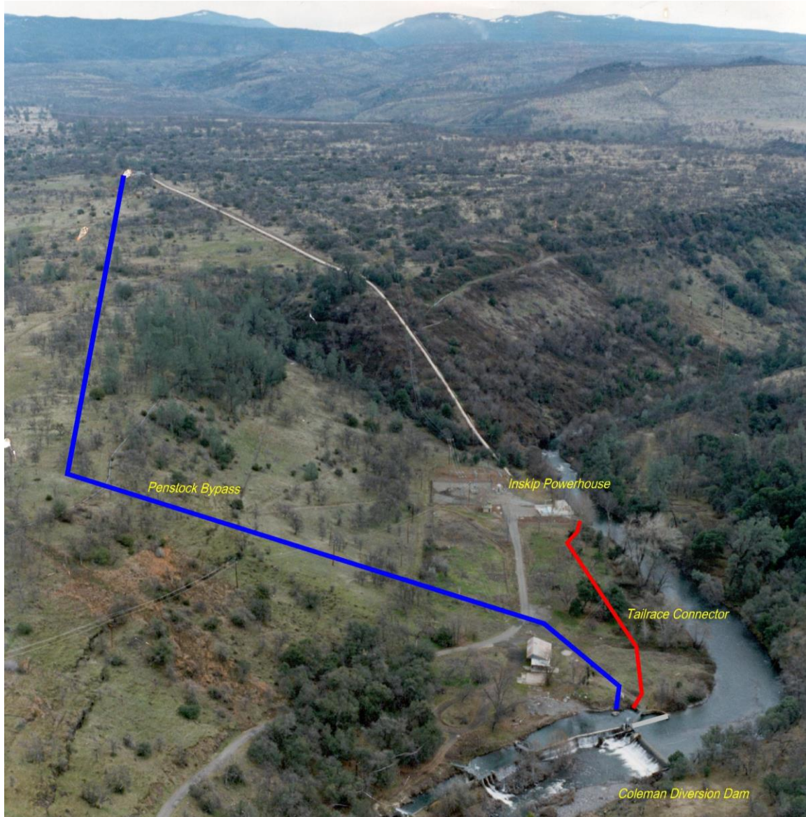
Before construction, ariel overview of the planned Inskip Powerhouse penstock bypass and tailrace connector, February 2007.
