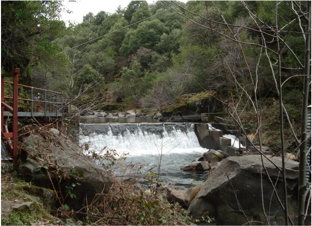
Before construction, photo of Wildcat Diversion Dam (center), February 2007.
