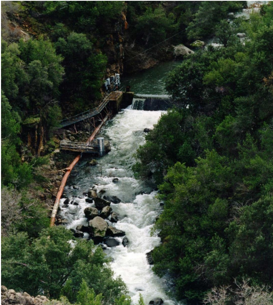
Before construction, photo of North Fork Battle Creek looking upstream at Wildcat Diversion Dam, June 2009.
