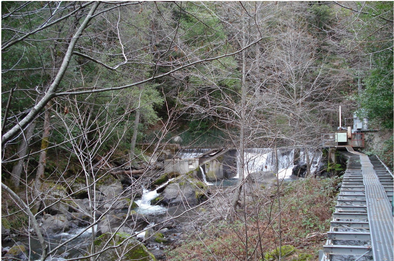
Before construction, looking upstream at the North Battle Creek Feeder Diversion Dam, the non-functioning fish ladder (center) and the unscreened diversion (right), February 2007.
