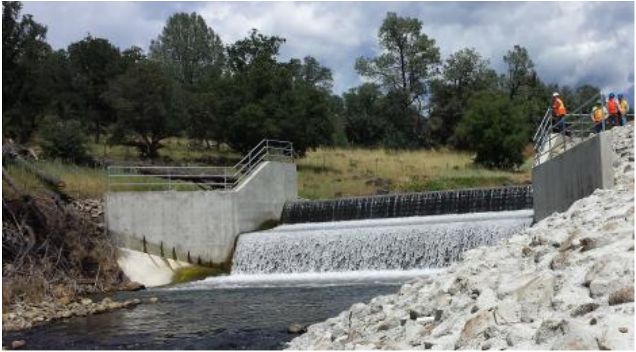
After construction, looking upstream at the new Baldwin Creek fish barrier weir, May 2014. The barrier weir acts as a jump barrier at low flows and a velocity barrier at higher flows to prevent anadromous fish from migrating upstream.
