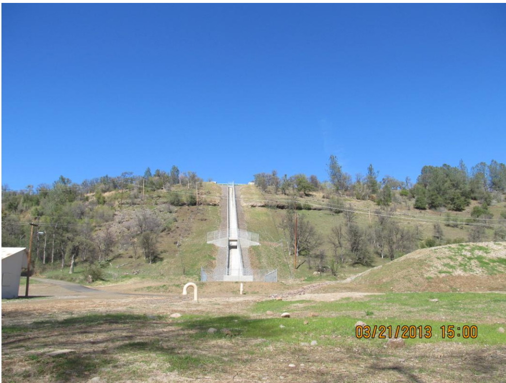
Coleman Diversion Dam/Inskip Powerhouse: Uphill view of the new penstock bypass chute and vegetation re-establishing in surround areas.
