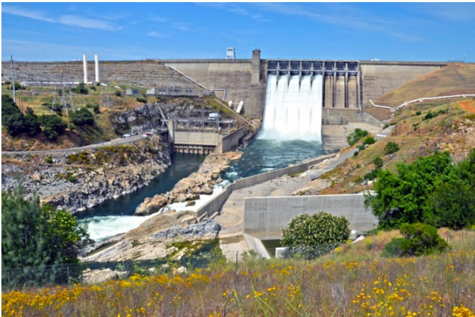
Folsom Dam with five gates open
