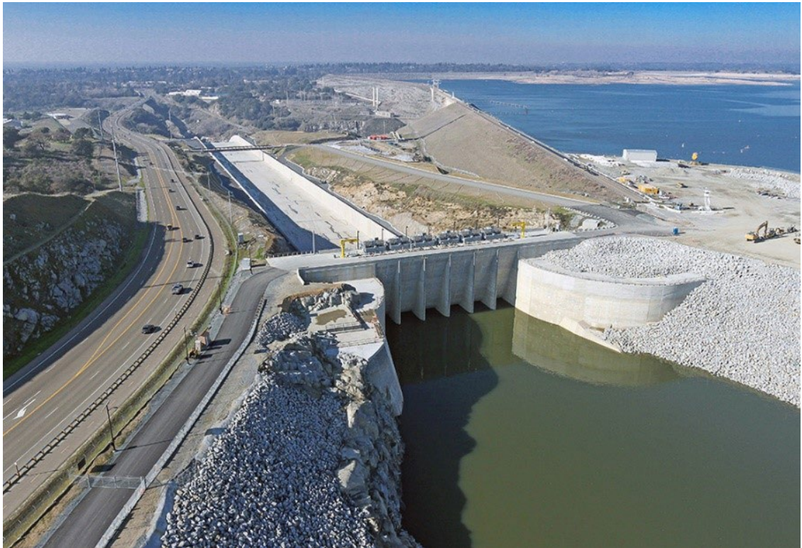
Photo illustrating Folsom Dam improvements and new auxiliary spillway.
