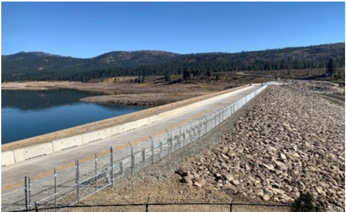
Photo showing completed dam modifications and reinforced road across Boca Dam.
