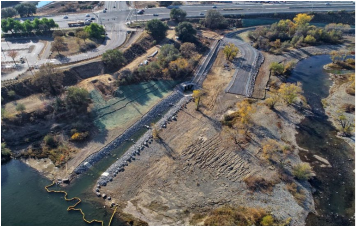
Aerial photo showing the new Nimbus Dam Fish Passage Project underway.
