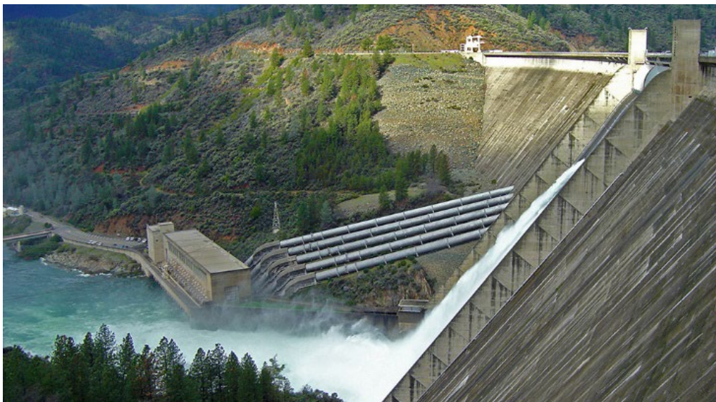
Shasta Dam shown above releasing 50,000 cfs of water.
