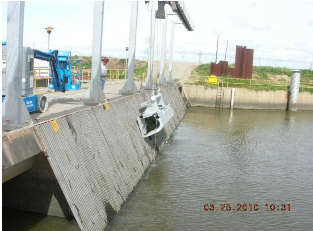
Figure H-1. Photograph of trash rack with 2 panels removed in spring 2010 (arrows indicate removed panels).
