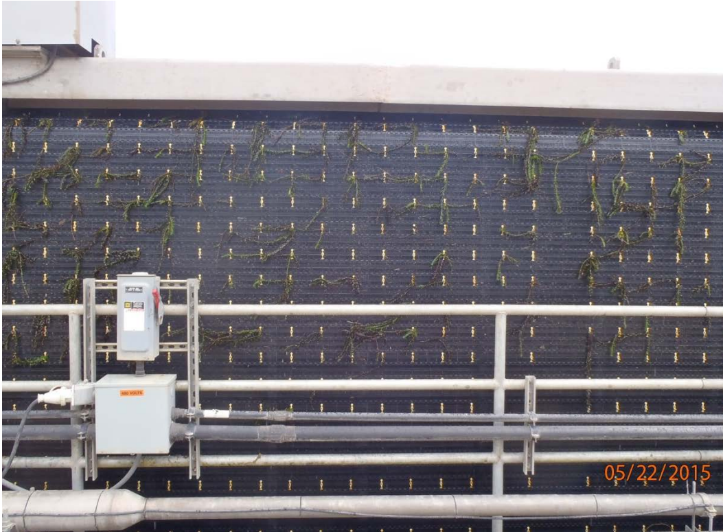
Figure 3. Debris pegs on the Hydrolox traveling screen loaded with the pond weed, Egeria.
