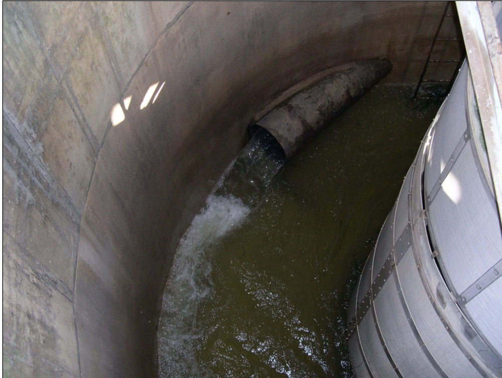
Figure 1. Holding tank (132,000-L, 35,000-gal), Tracy Fish Collection Facility, Byron, California.
