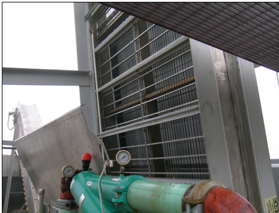
Figure 2a.—Vertical traveling screen out of the water (control condition).
