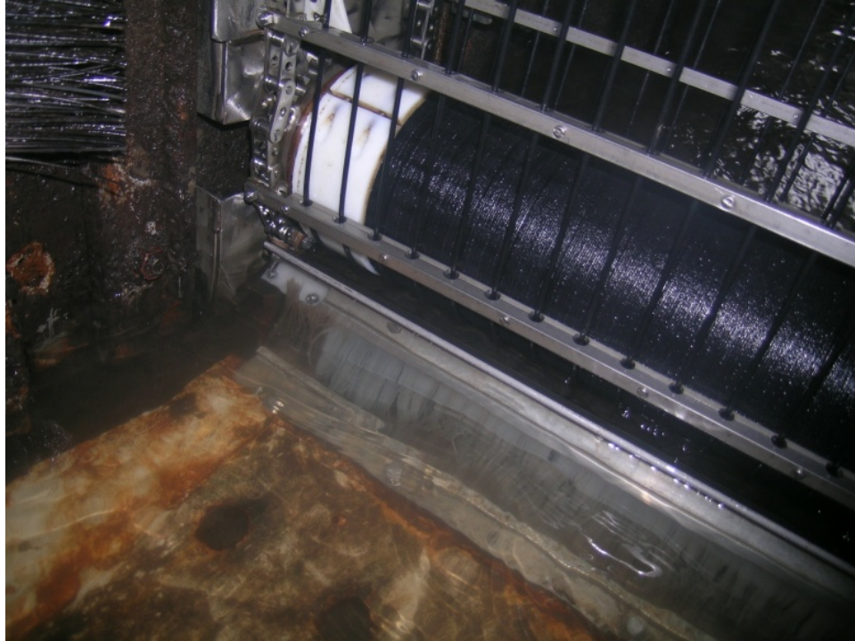
Figure 2b.—Vertical traveling screen all the way down, steel plate flat (plant condition).
