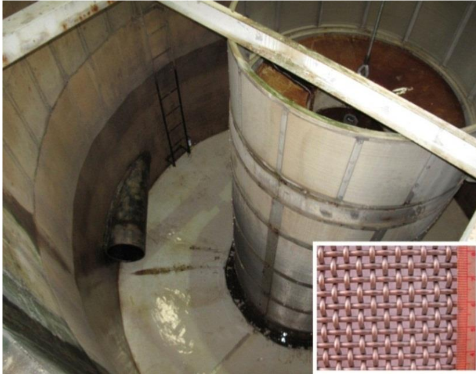
Figure 1.—Holding tank screen at the Tracy Fish Collection Facility (Bureau of Reclamation, Byron, California) that was tested to determine retention efficiency of 20–30 mm FL juvenile delta smelt during 30-minute collection periods. Inset: Close-up of holding tank screen material (average wire diameter = 2.1 mm, average square opening = 2.7 mm, average diagonal opening = 3.8 mm; figure from Reyes et al. 2012).
