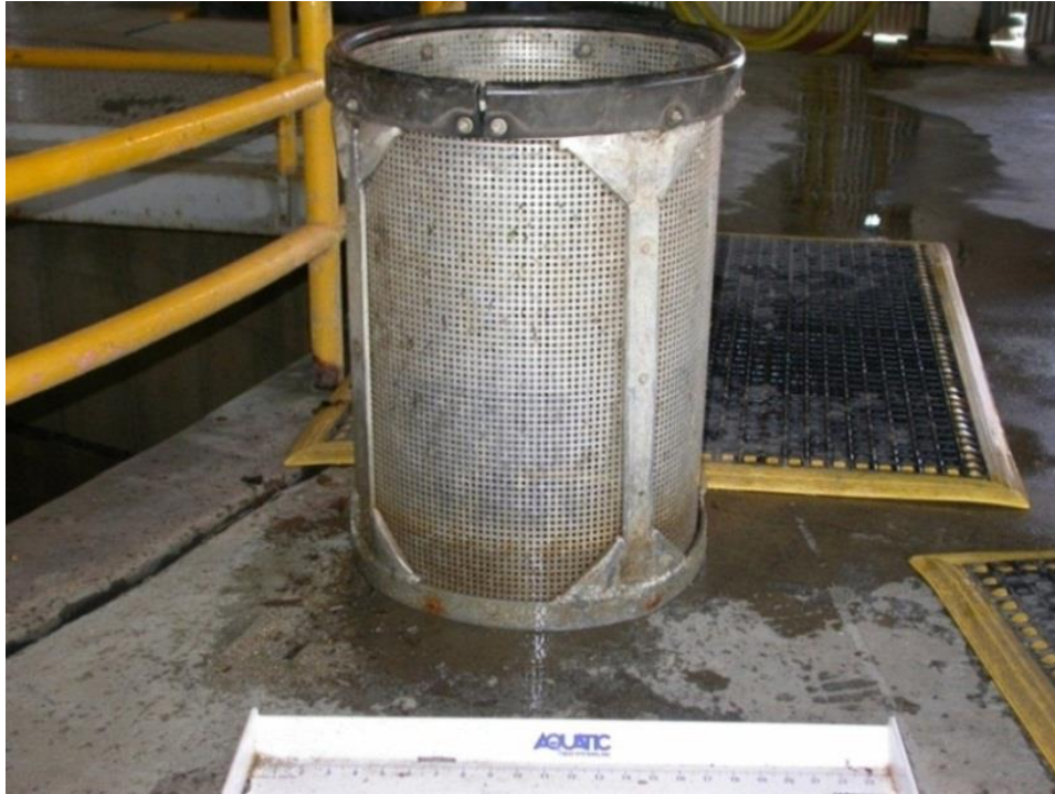
Figure 2.—Fish count station screen (maximum circular hole diameter = 4.8 mm) at the Tracy Fish Collection Facility (Bureau of Reclamation, Byron, California) that was tested to determine effectiveness at retaining juvenile delta smelt in 2004 and 2005 by Sutphin et al. 2007.
