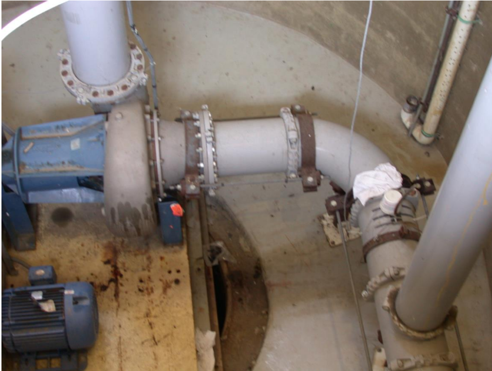
Figure 2.—Hidrostal pump used to transfer adult and juvenile delta smelt ( Hypomesus transpacificus ) from the secondary channel into a receiving pool at the Tracy Fish Collection Facility (Byron, CA) where they could be captured and processed to evaluate secondary channel louver efficiency and louver participation.
