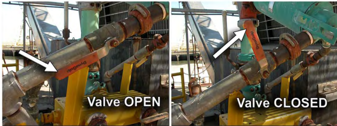
FIGURE 14.—Closeup of the DynaQuip valve showing OPEN and CLOSED valve positions. All valves operate similarly.
