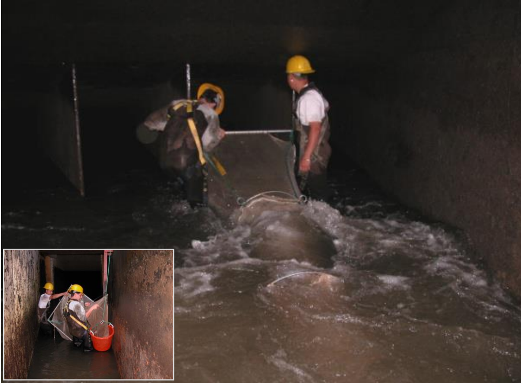
Figure 5.—Modified fyke net being used to remove predators from bypass 2 in the Tracy Fish Collection Facility secondary channel. Fish were removed from randomly selected bypass tubes by increasing water velocities in the tube to flush out fish. Inset: Fish were emptied into a plastic basket and lifted out of the secondary channel.
