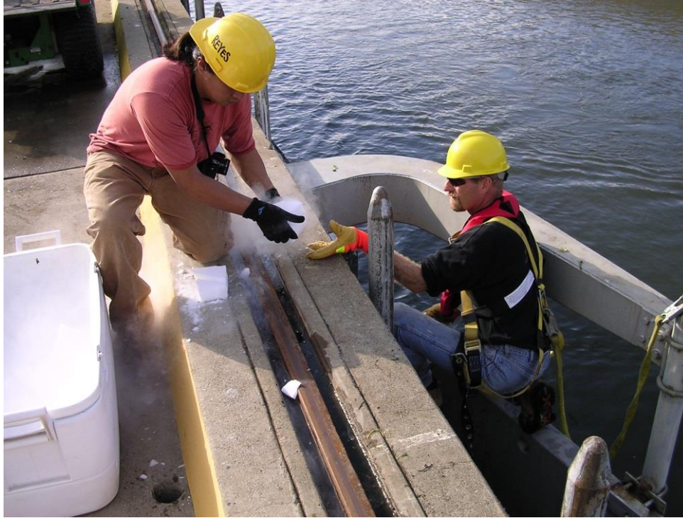
Figure 5.—Team of 2 people inserting dry ice into bypass tube opening at the Tracy Fish Collection Facility. The bypass tube leads to the secondary channel which directs fish to a holding tank. Dry ice was inserted to move fish from the bypass tubes and secondary channel into a holding tank.
