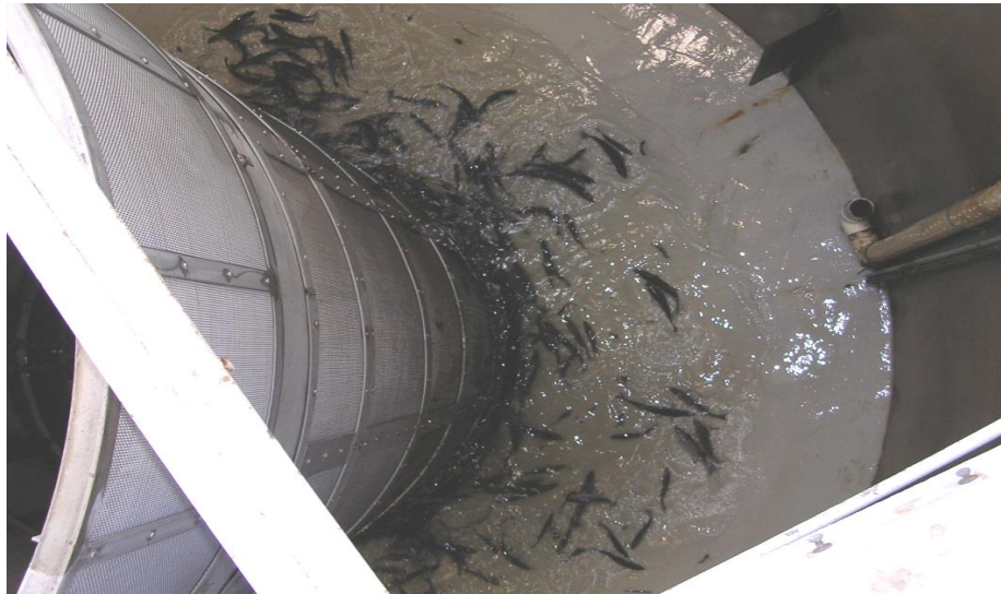
Figure 24.—After carbon dioxide treatment (349 mg/L peak carbon dioxide concentration), fish were forced from the secondary channel (top) into the holding tank (bottom).
