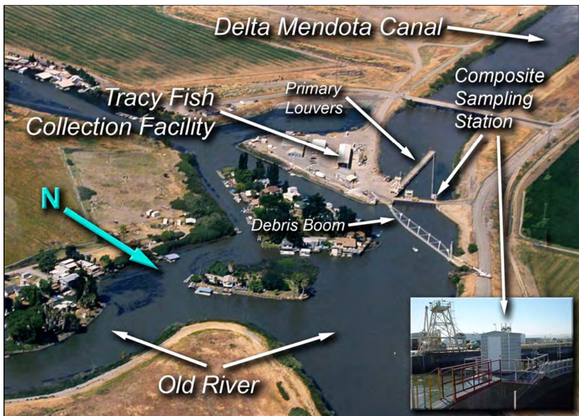
FIGURE 2.—Aerial photograph showing the Tracy Fish Collection Facility and the location used for the composite sampling. The calibration shed used to house the composite sampling pumps is shown in the inset. Reclamation photographs.
