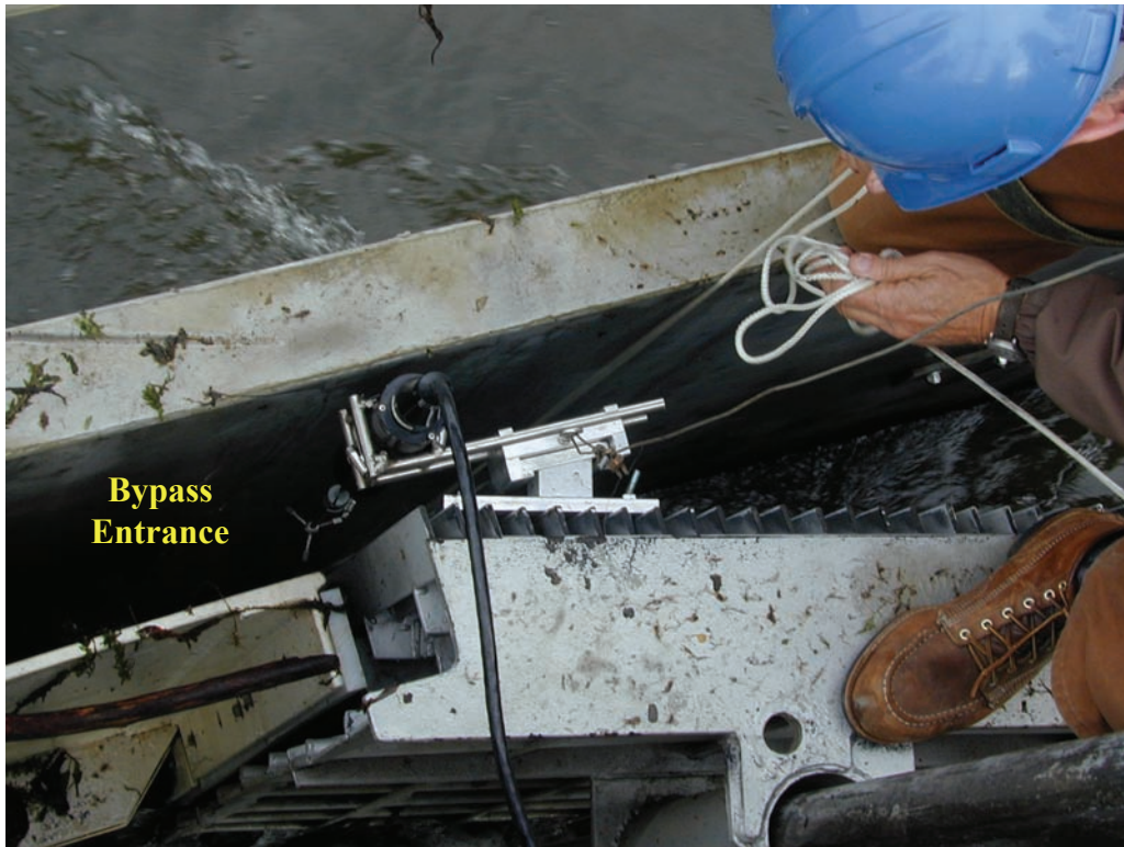
FIGURE 7.—The ADV was lowered down on the deployment rail into the bypass entrance.
