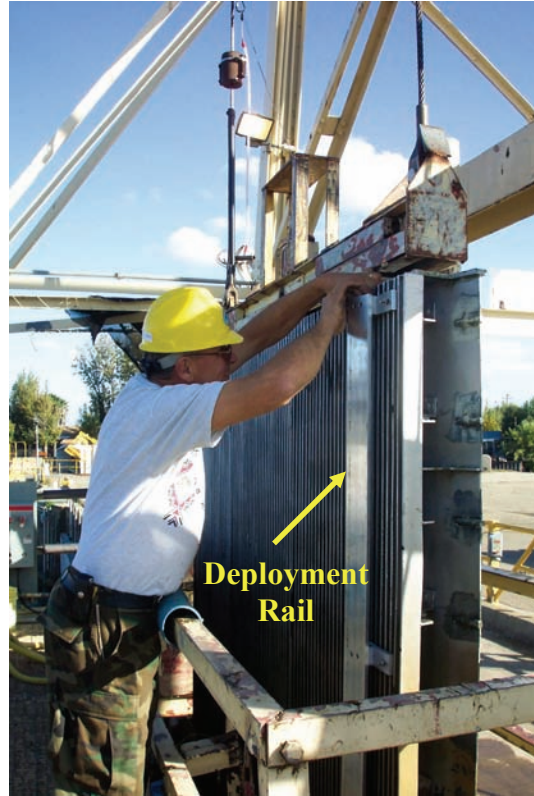
FIGURE 5.—An ADV deployment rail was affixed to the louver panel just upstream from the bypass entrance.
