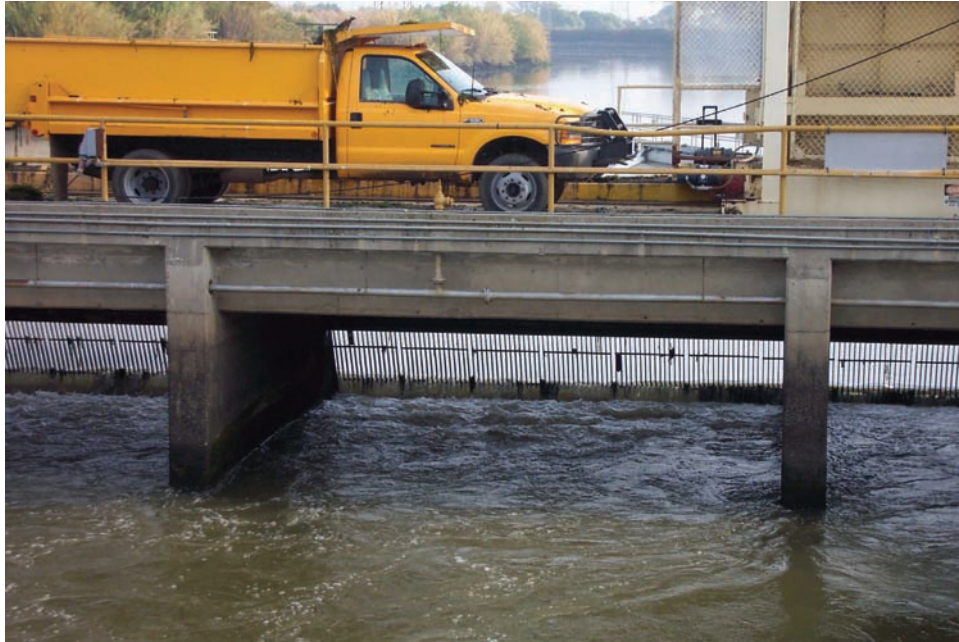
FIGURE 12.—Trashrack fouling was documented during data collection.
