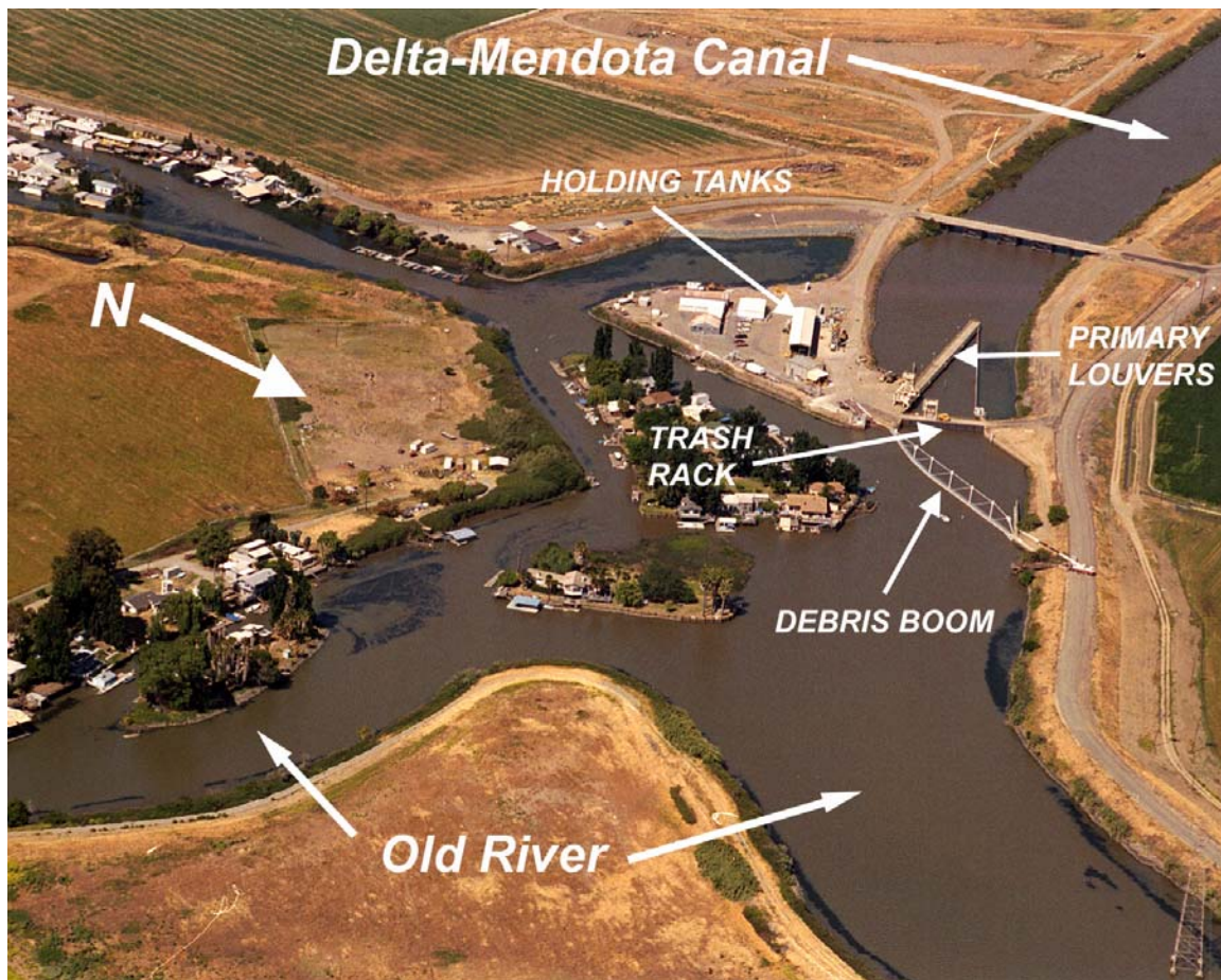
FIGURE 1.—Tracy Fish Collection Facility, Old River Branch of the San Joaquin River, California.
