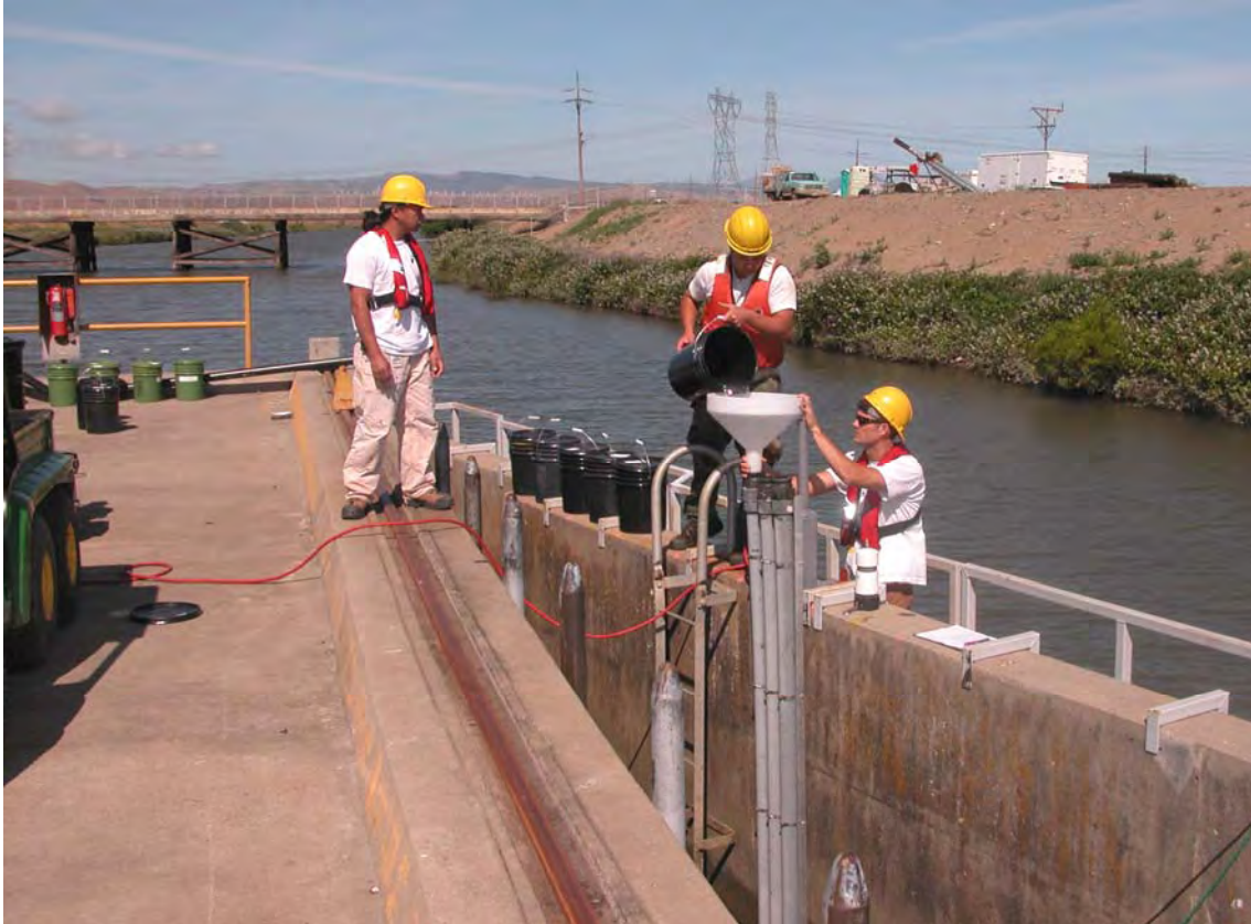
FIGURE 4.—Reclamation fishery biologists transferring Chinook salmon into insertion tubes in front of bypass No. 4 at the Tracy Fish Collection Facility.
