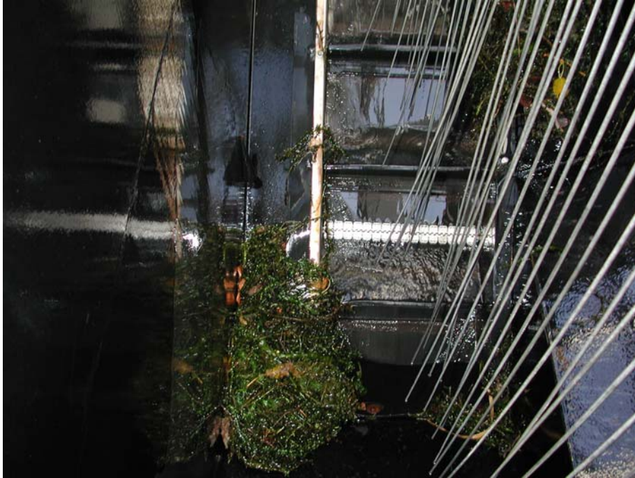
FIGURE 3a.—Before: At the back wall of the hopper (west ledge) debris too large to flow through the drain tube would accumulate at the base of the hopper.
