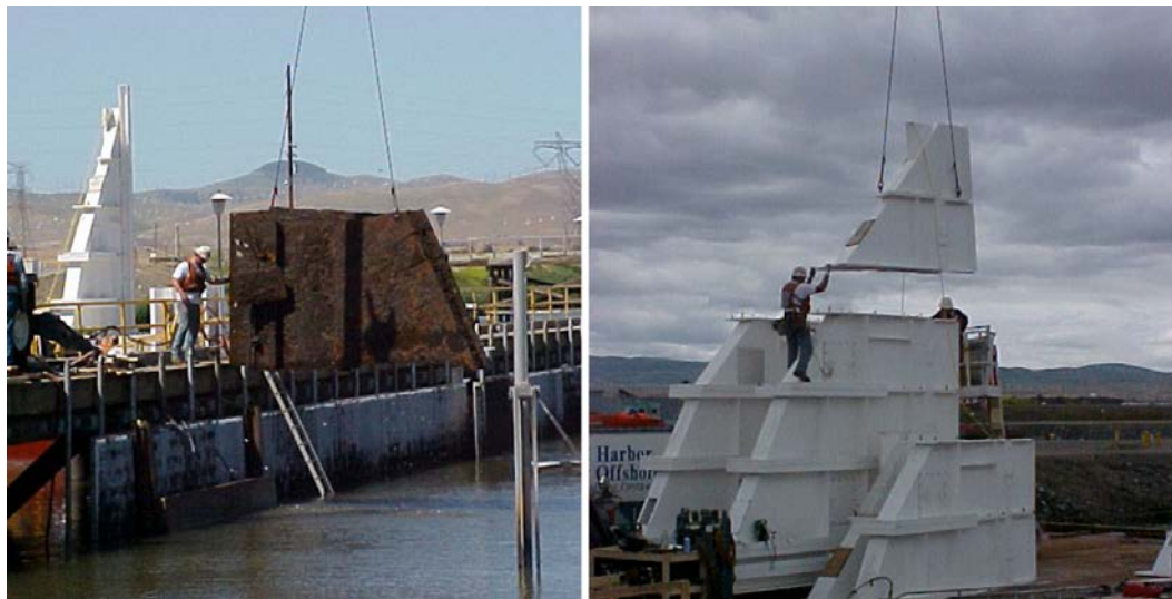
Figure 13 Transition boxes replacement at the Tracy Fish Collection Facility
