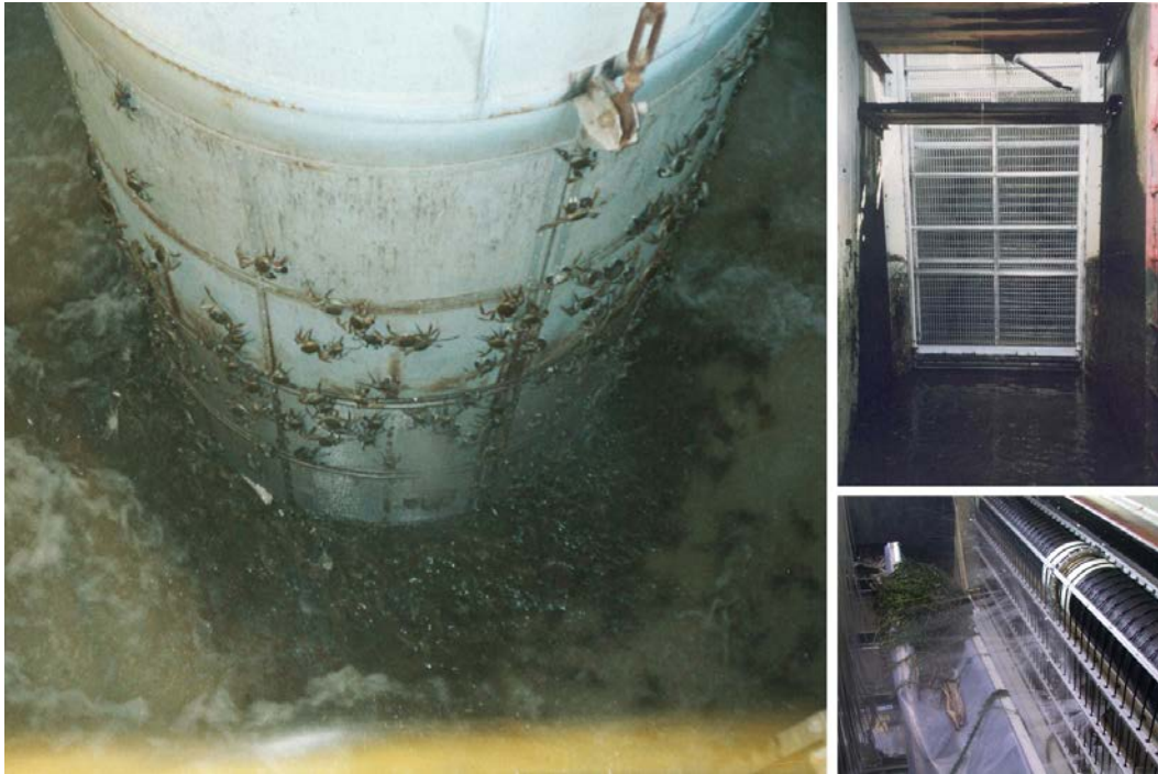
Inset: Traveling screen installed upstream of the secondary louvers (top) and high-pressure spray to wash mitten crabs off the traveling screen (bottom).
