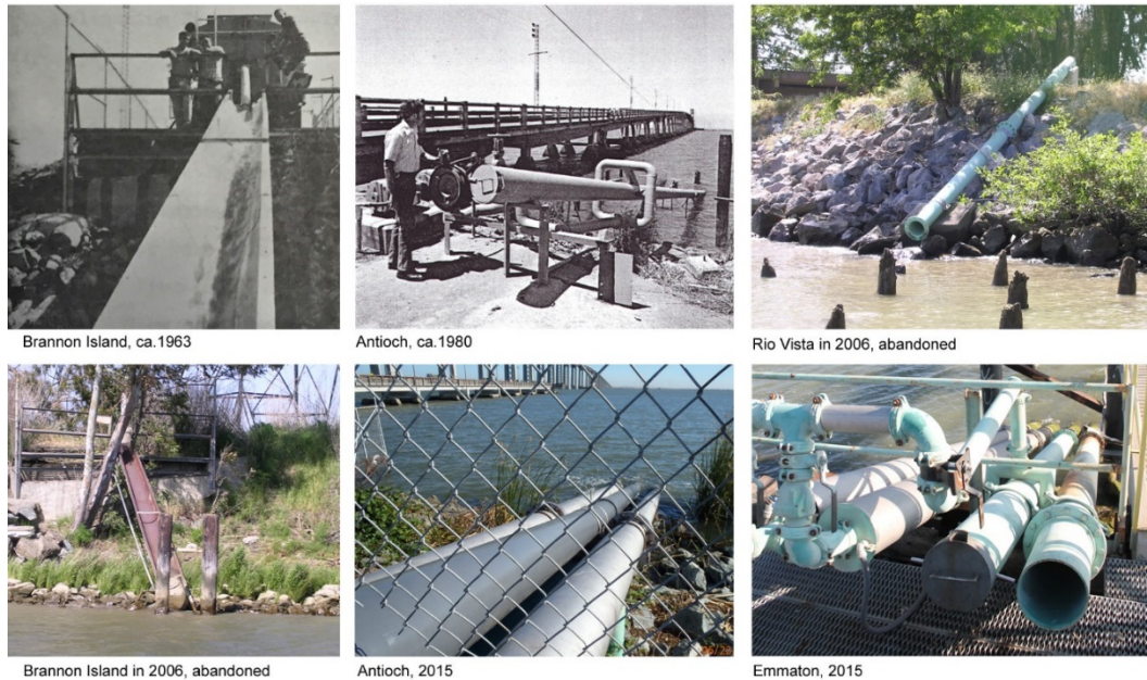
Note: From left to right: Brannon Island site showing “dumping chutes” ca. 1963, Brannon Island site in 2006, Antioch site ca. 1980 with a single release pipe, Antioch site in 2015 with the additional flushing assembly (note the gradual slope of the pipes), incomplete Rio Vista site in 2006, and the Emmaton site in 2015 (note steep slope of the pipes).
