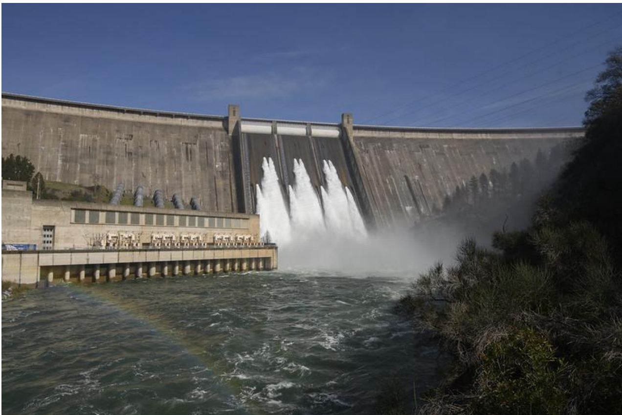
Cover Photo: Shasta Dam releasing storage after storm, February 2022. (Reclamation)
