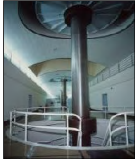
The Davis Dam Powerplant is linked with a Federal power distribution system operated by the Western Area Power Administration. The total system consists of 2,100 miles of high-voltage transmission lines serving 43 power substations in Arizona, Nevada, and California.
