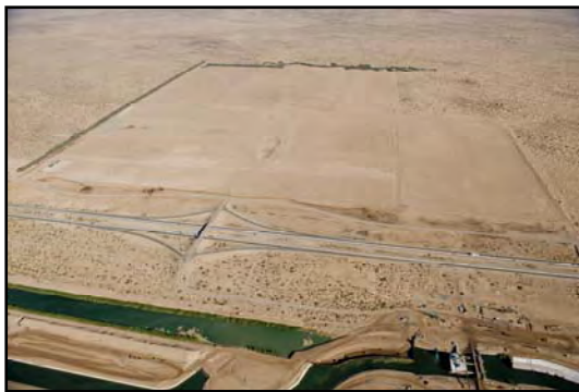
Drop 2 Storage Reservoir Project will provide more capacity for water storage in the Colorado River below Parker Dam.
