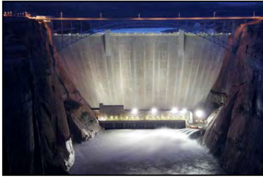
Glen Canyon jet bypass tubes releasing water during the high-flow experiment, which was also intended to supply sand needed to protect archaeological sites and create backwaters used by young native fishes, particularly endangered humpback chub.
