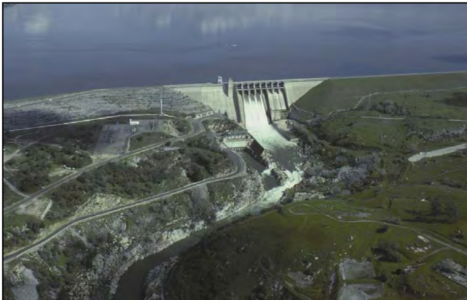
Reclamation installed integrated security systems at Folsom Dam.
