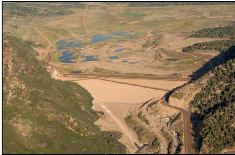
Aerial view of Ridges Basin Dam construction.
