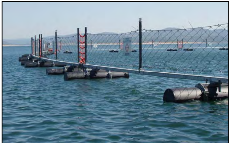
Boat barriers at Folsom Dam.
