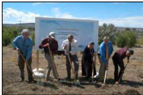
Reclamation awarded a $4.6 million contract to begin construction of the Navajo Nation Municipal Pipeline.
