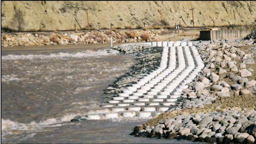
The completed Price-Stubb fish passage allows upstream migration of fish.
