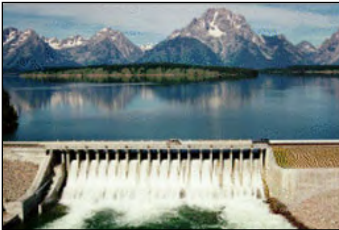
Reclamation will emphasize water management planning under the Water for America Initiative through its Investigations Program and the introduction of a new Basin Studies Program. Photo shows Jackson Lake Dam in northern Wyoming.
