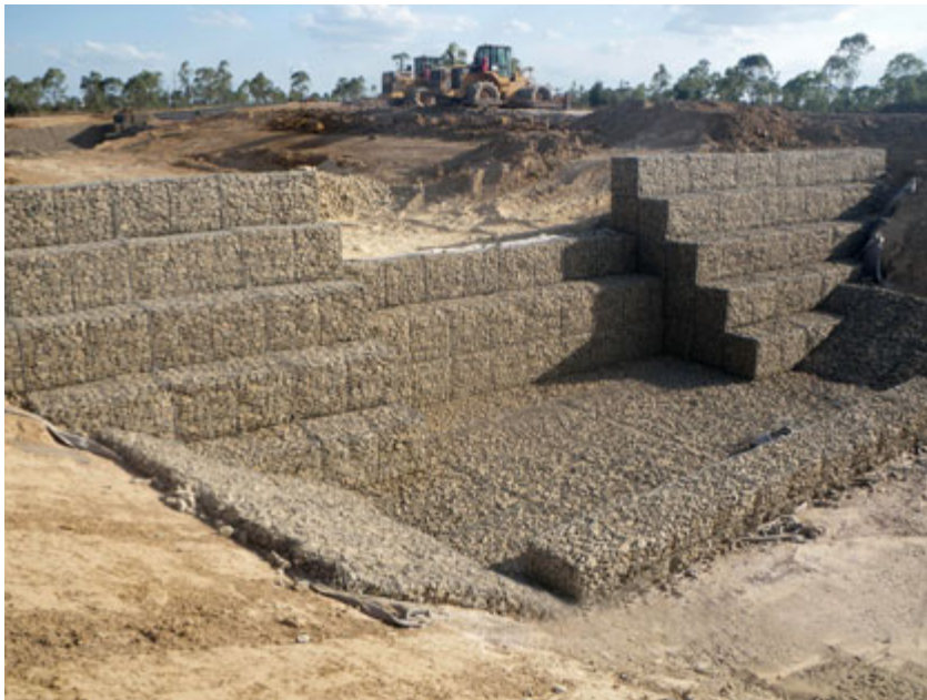
Photo 17. Gabion check dam in Moranbah, Queensland, Australia. Notice the Reno-mattress placed downstream of the check structure for scour protection. Photo by Prospect Contractors, Australia. http://www.prospectcontractors.com.au/anglo_coal.html
