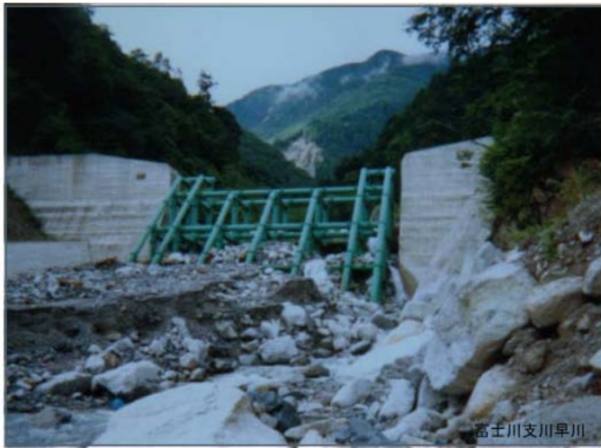
Photo 16. Open grid-type check dam
