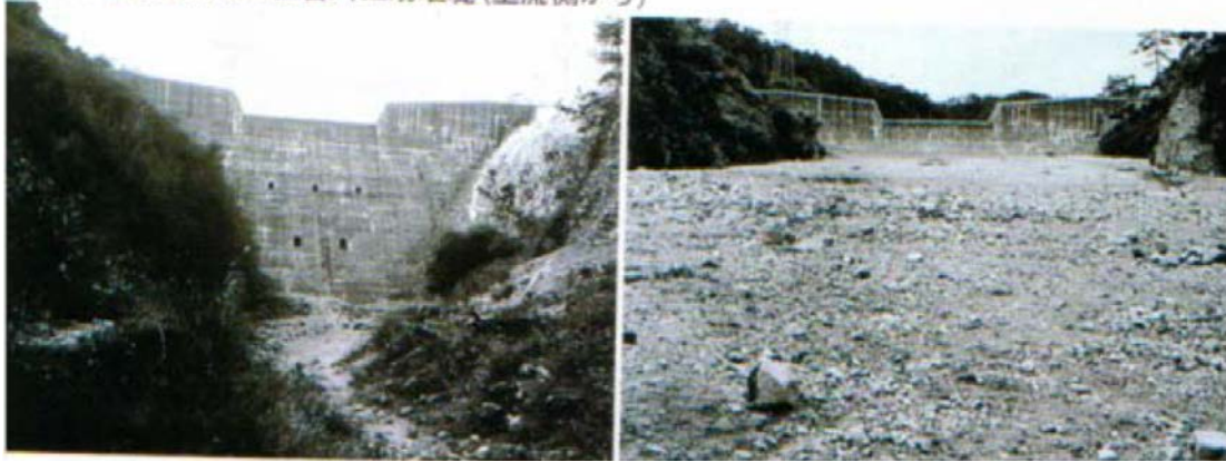
Photo 14. Closed-type concrete check dam in Sumiyoshi River, Rokko Mountain, Japan, 1967. Source: Mizuyama, T (2008) Structural Countermeasures for Debris Flow Disasters
