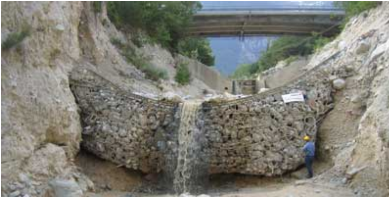
Photo 12. A flexible ring-net barrier that is impounding debris. Notice the sediment laden water that is passing through the structure. Source: http://www.geobrugg.com
