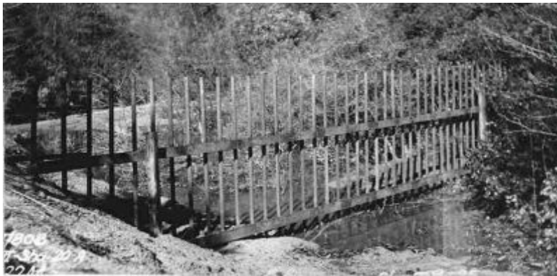
Photo 11. A debris rack/fence (no fence fabric) used to capture material upstream of a culvert. Photo courtesy of the Federal Highway Administration.
