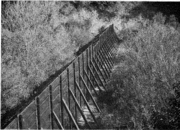
Photo 13: Debris Barrier Wall in Southern California. Source: USACE (1993) Assessment of Structural Flood-Control Measures on Alluvial Fans
