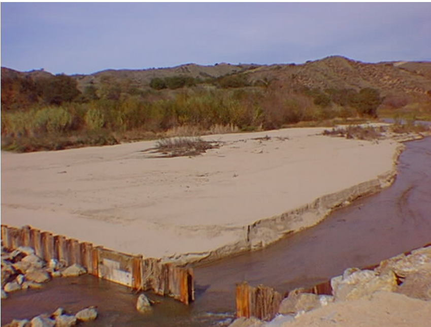
Photo 5 - Existing sheet pile dam, photo date unknown. Note left most stoplog slot has logs removed. Water is cutting through accumulated sediments. The stoplog appears to have been removed after the sediment deposition. Compare this photograph to photograph numbers 1 and 2 where vegetation growth covers and conceals sediment deposits.
