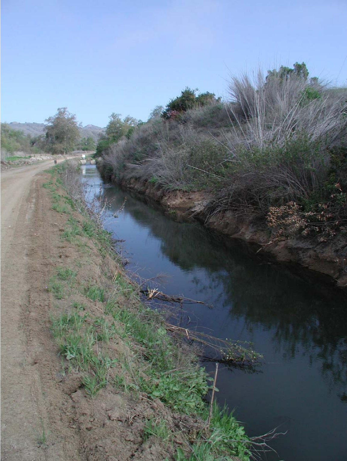
Photo 3 - Existing O'Neill ditch with headworks around the distant corner, March 2004. Parshall Flume near the photo top used for flow measurement.
