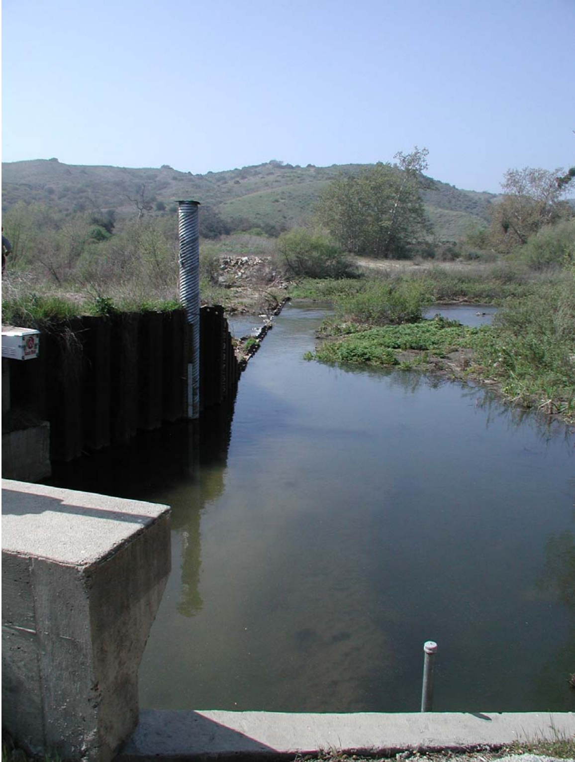
Photo 6 - Existing sheet pile dam, March 2004. View off headworks top. Note the sediment accumulating just below water surface near the diversion intake.
