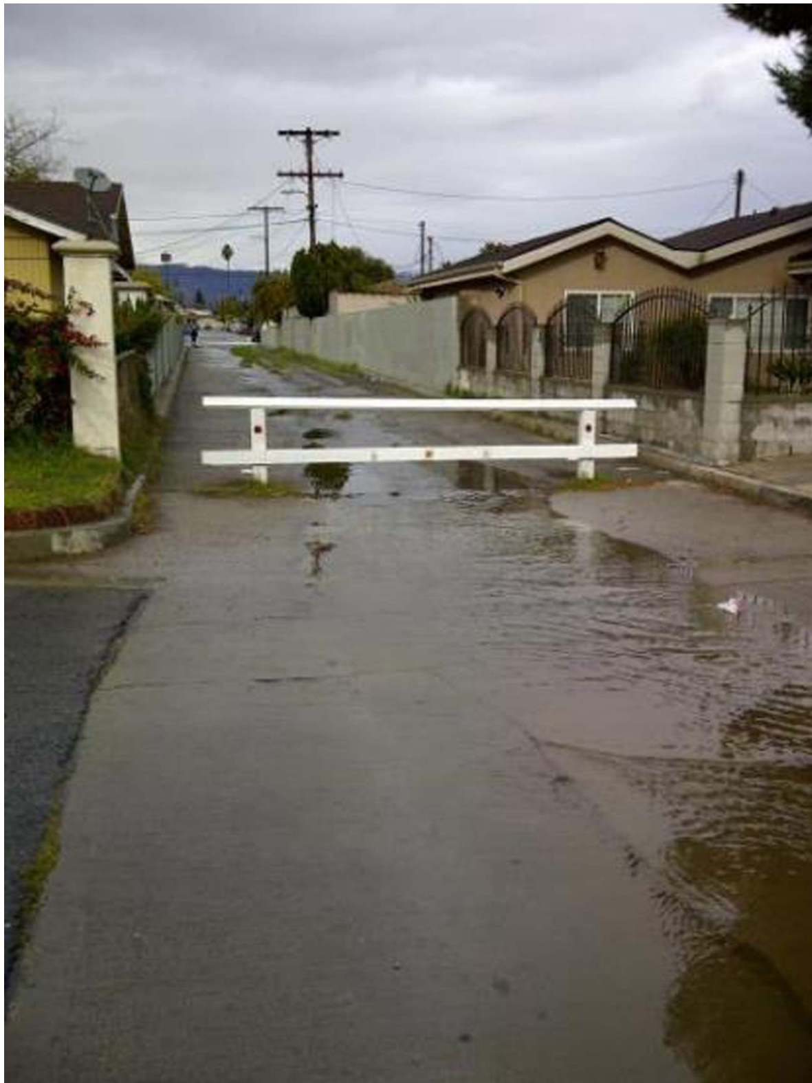
Figure 1 - Paseo South Entrance Before Project
