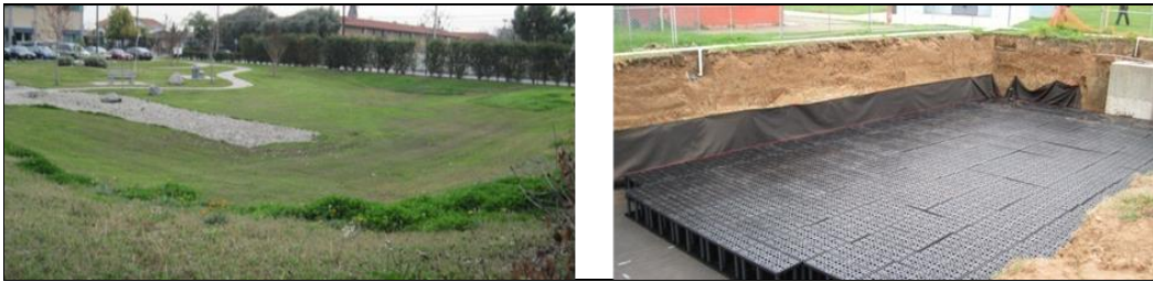
Figure 7. Surface Infiltration Basin and Underground Infiltration Chambers
