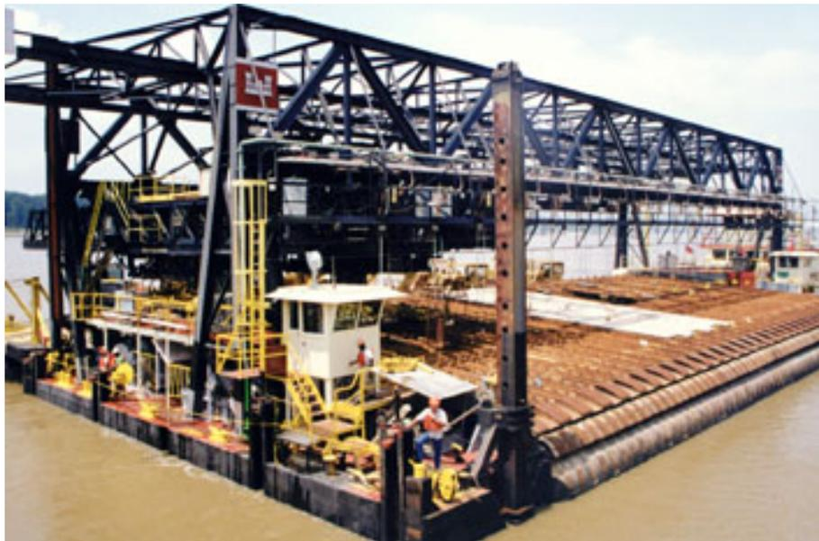
Photo 5: Barge used to Deploy Prefabricated Scour Protection in Mississippi River
