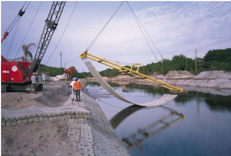
Photo 4: Deployment of Prefabricated Armoring in Canal
