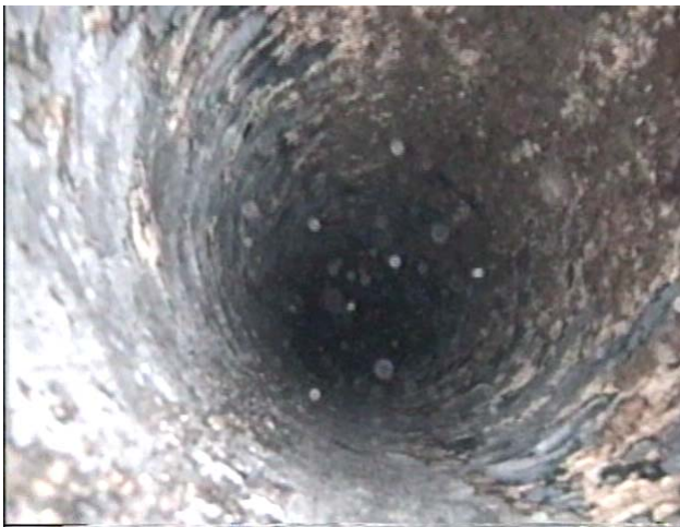
Figure 3. 10-in domestic water line before and after water jetting.
