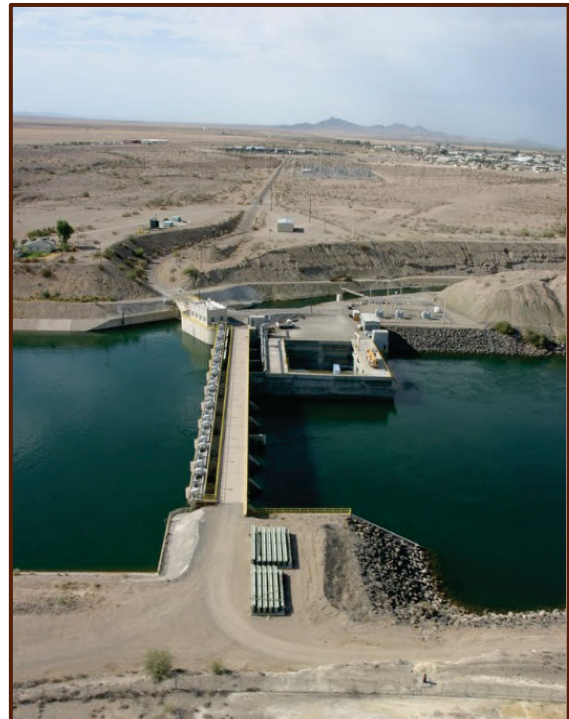
Headgate Rock Dam - forms Lake Moovalya, houses 18MW hydro powerplant, and serves as an entry gate to the Colorado River Irrigation Project.
