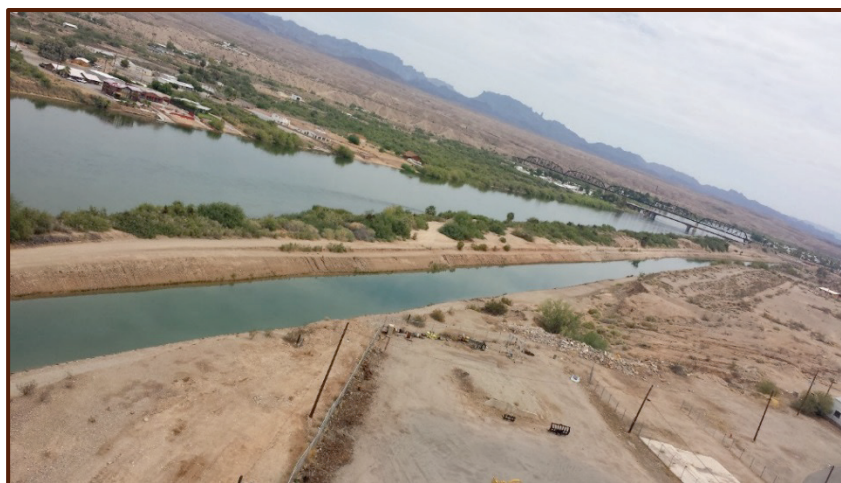
Unlined section of Main Canal - example of older construction methods and area of potential improvement.
