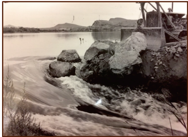
Bulldozer pushes boulder into breach, closing last remaining channel creating Lake Moovalya behind Headgate Rock Dam. Date: 11/08/1940.
