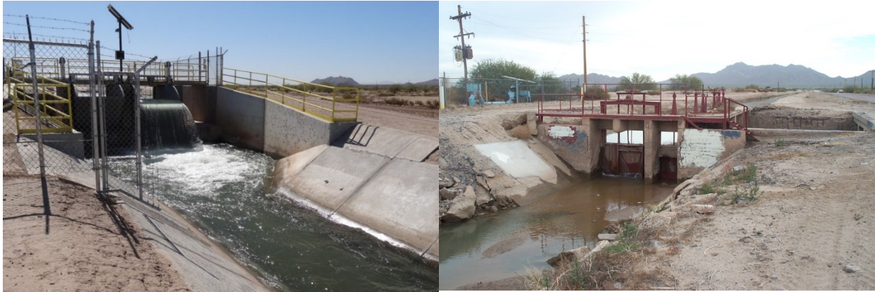
Figure 4 Photo of an Automated Drop Control Structure on the Reconstructed Casa Blanca Canal (Left; Credit: B. Barker, May 24, 2021); and Photo of the Casa Blanca Canal Headworks and Unlined Pima Canal Before Improvements (Right; Courtesy of David DeJong, 2006).
