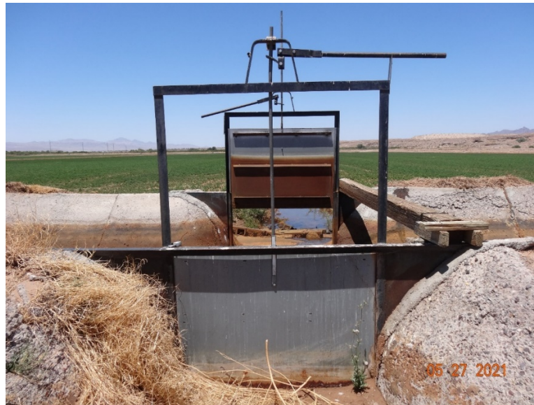
Figure 40 Photo of a Locked and Sealed Field Turnout Gate Serving a Fallowed Field in the Mohave Valley Irrigation District (credit: B. Barker, May 27, 2021).
