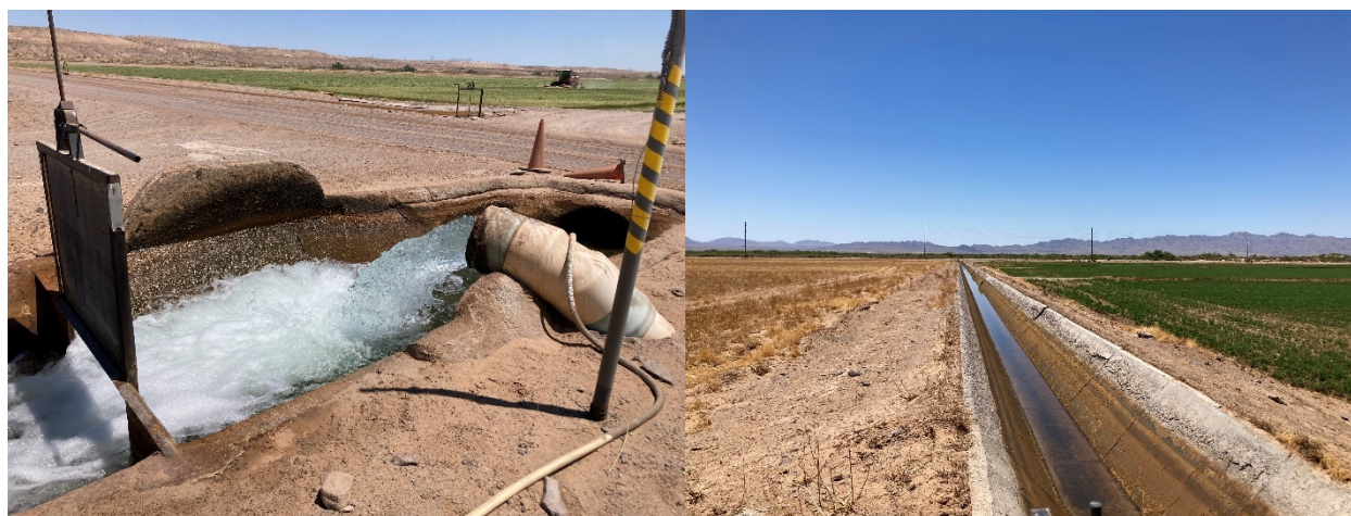
Figure 38 Photos of Irrigation Infrastructure in the Mohave Valley Irrigation District (credit: L. Perkins, May 27, 2021).
