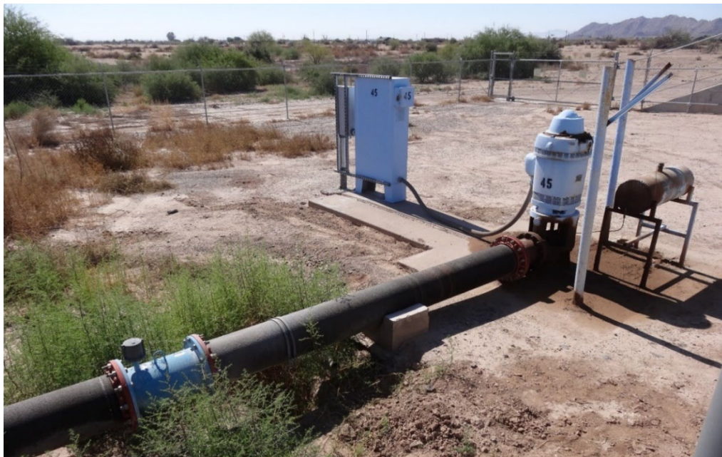
Figure 5 Photo of an Irrigation Supply Well for the Pima Canal with a Flow Meter Installed in the Discharge Pipe (Credit: B. Barker, May 24, 2021).
