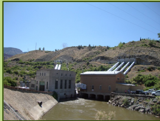
Orchard Mesa Pumping Plant
