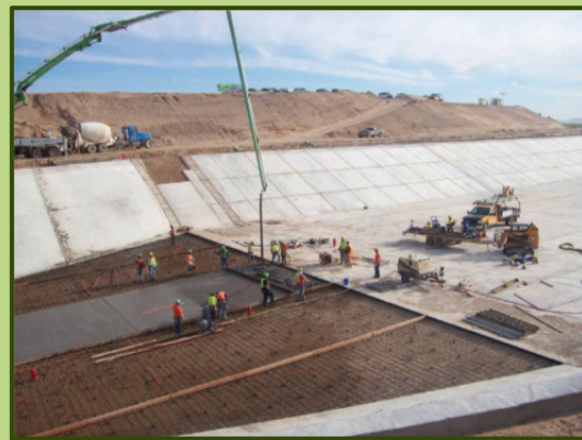
All-American Canal lining in progress Used by permission of IID
