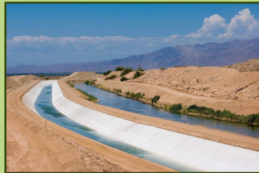
Water begins to flow through the new canal adjacent to the original earthen structure
