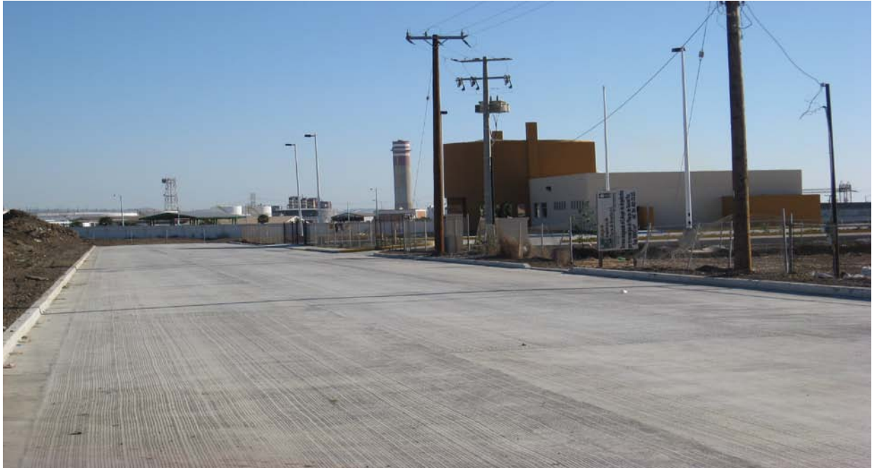
Figure 2-4: Between S5 and S6-Civil Engineering Society Building
