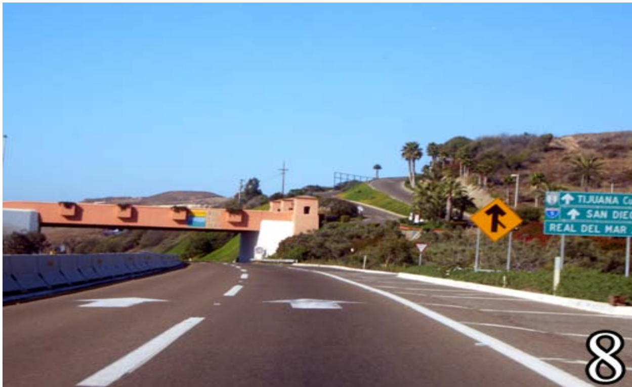
Grade Separation at Real del Mar
