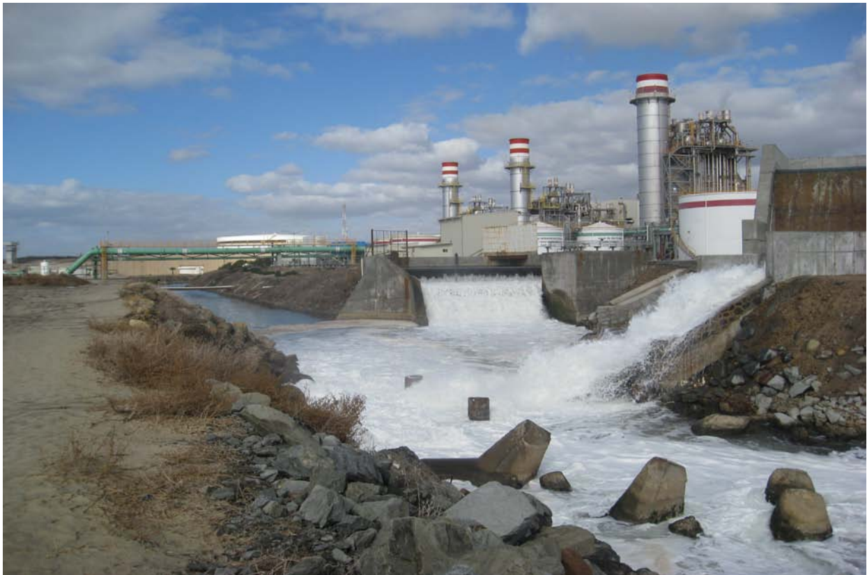
Figure 2-5: CFE Power Plant Outfall
