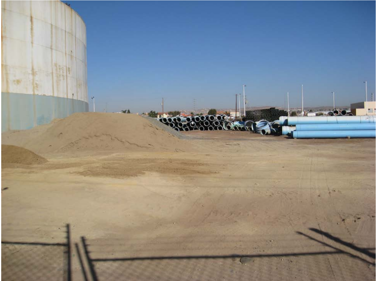
Figure 2-3: Site S6-Tanks and Maintenance Area
