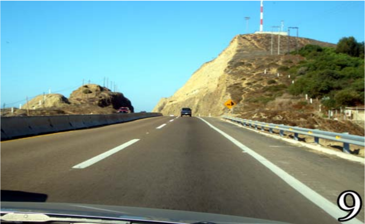
Steep Cut Slopes
