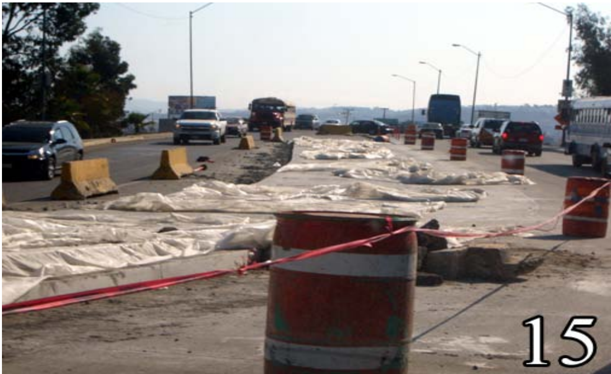
Construction of 8" PCC Overlay
