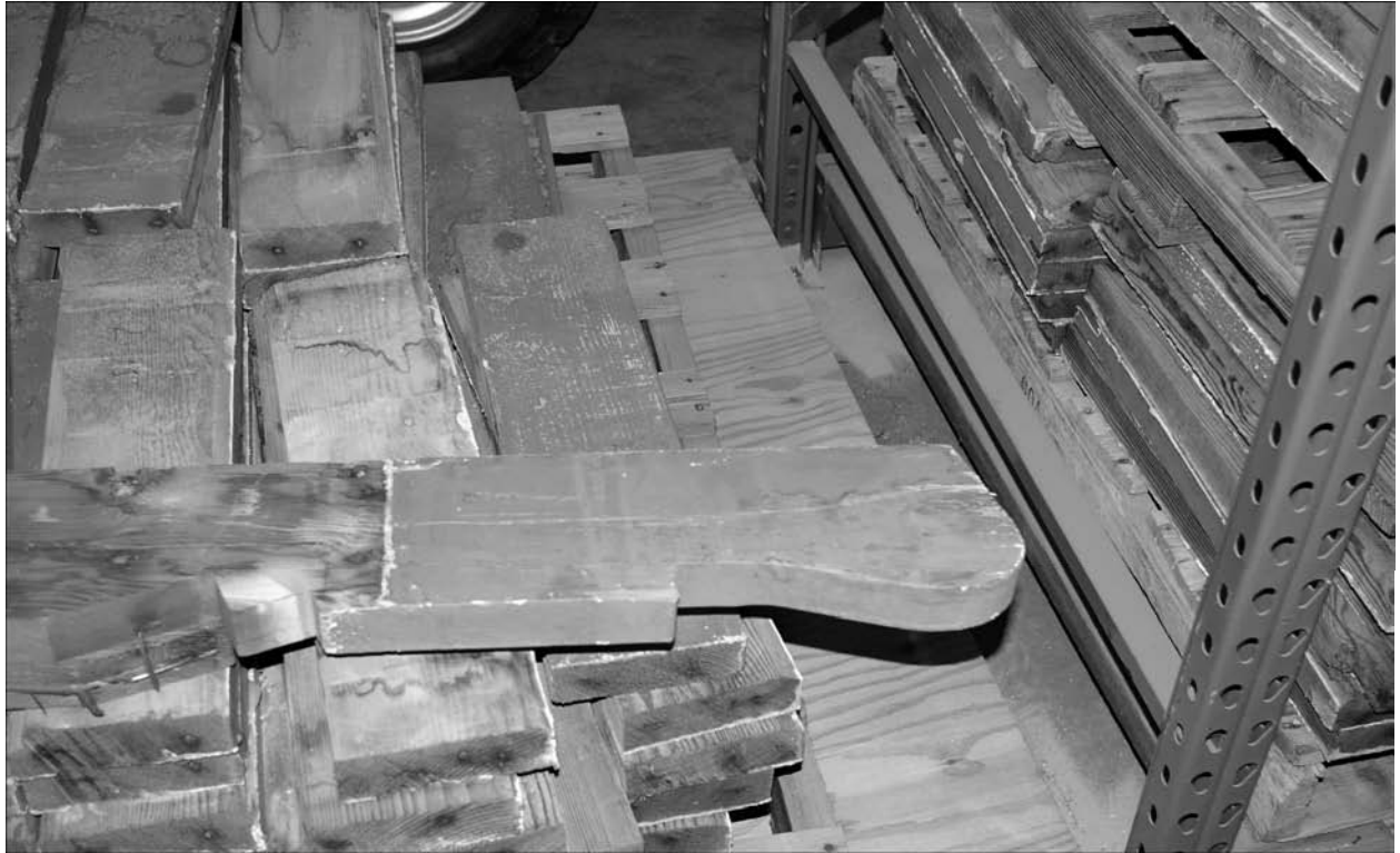
Figure 16. Faux rafter tails and associated blocking in storage, February 2009.
