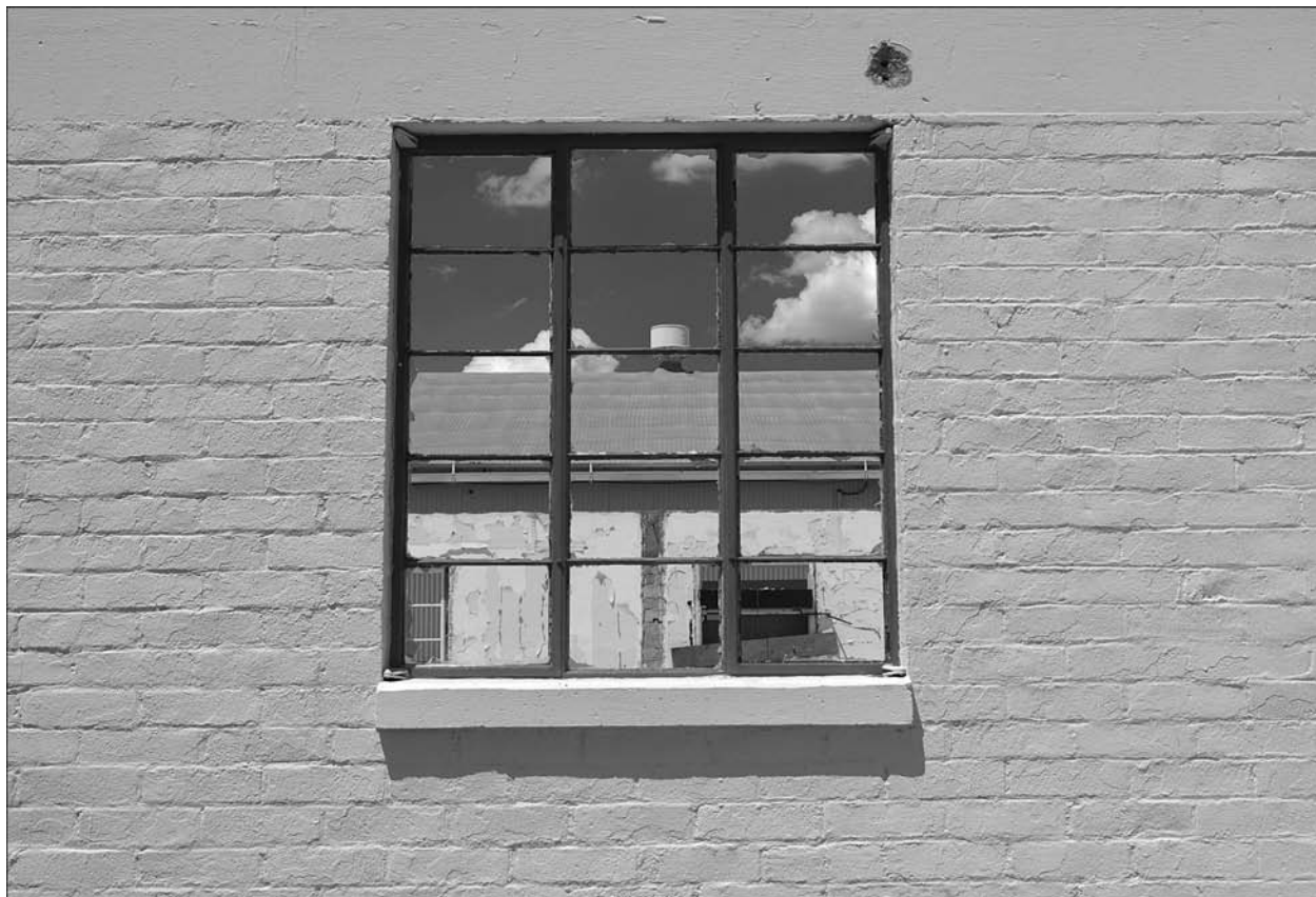
Figure 7. Fifteen-light, paired steel-sash casement window (exterior of Window 17), August 2007.
