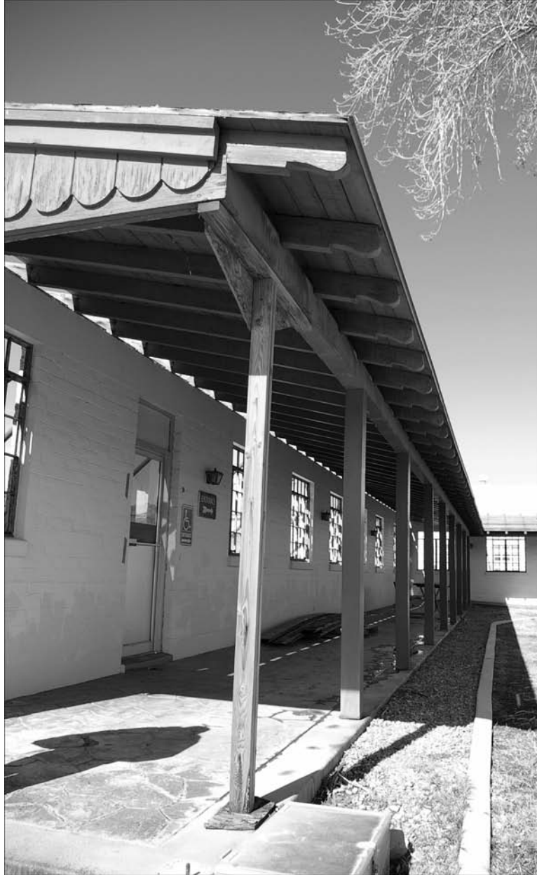
Figure 15. Temporary post in walkway covering, February 2009.
