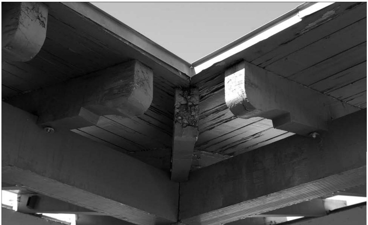
Figure 14. Example of mildew on rafter tail of walkway covering, February 2009.
