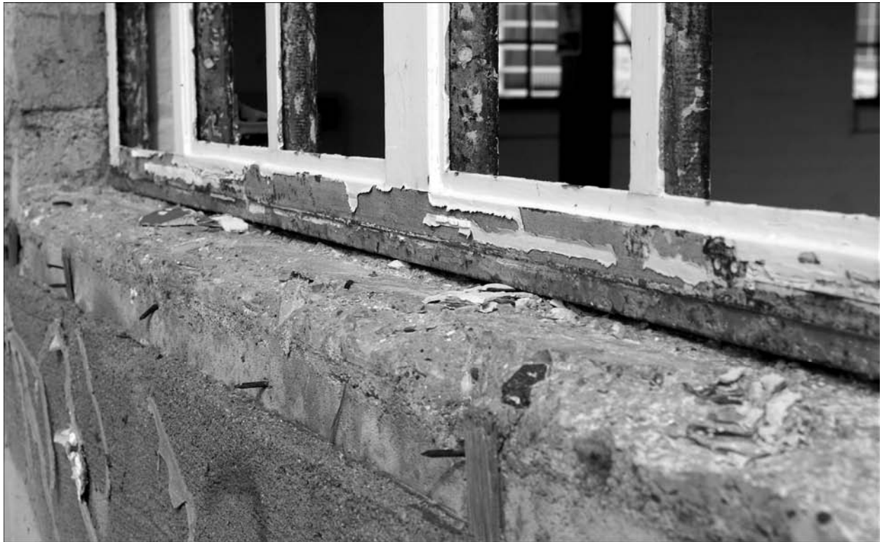
Figure 11. Example of minimal corrosion (interior of Window 2), February 2009.
