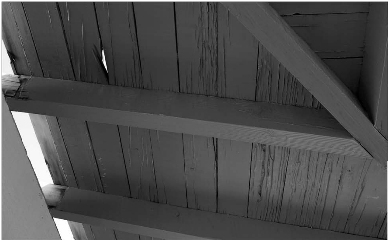
Figure 13. Example of peeling and cracking paint on underside of walkway covering, February 2009.
