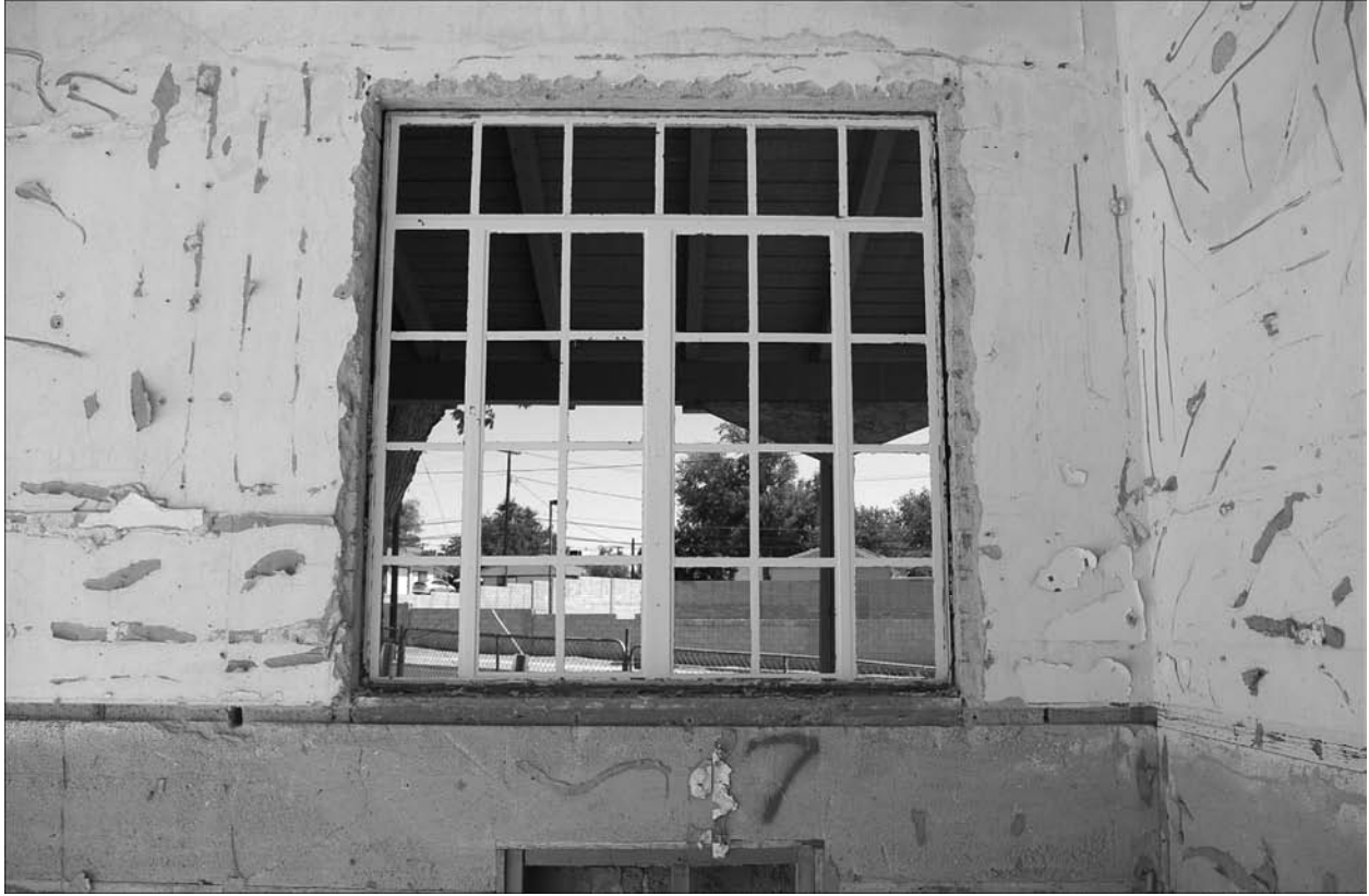
Figure 6. Thirty-light, paired steel-sash casement window (interior of Window 7), August 2007.
