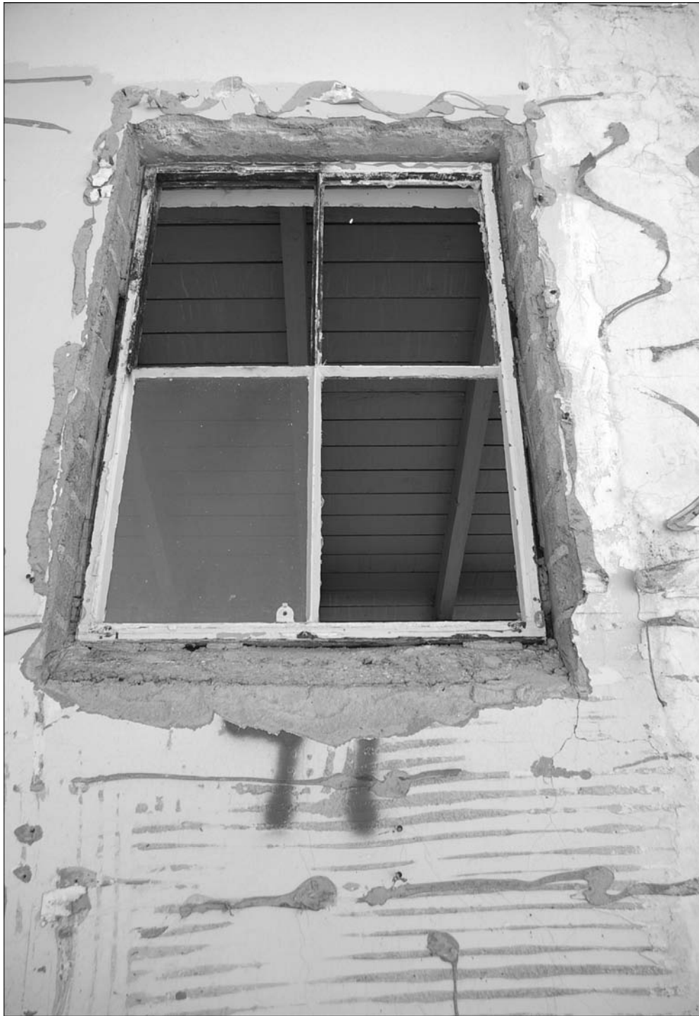
Figure 9. Four-light, steel-sash pivot window (interior of Window 41), August 2007.
