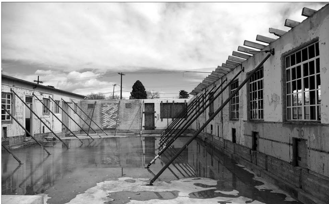
Figure 4. Interior of east wing showing steel support beams bracing the walls, February 2009.
