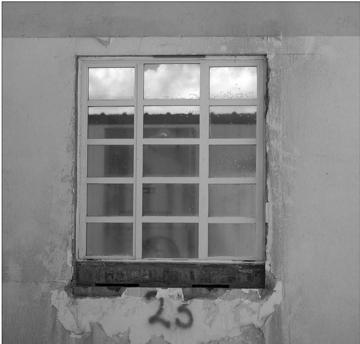
Figure 10. Fifteen-light, paired aluminum-sash casement window (interior of Window 23), August 2007.
