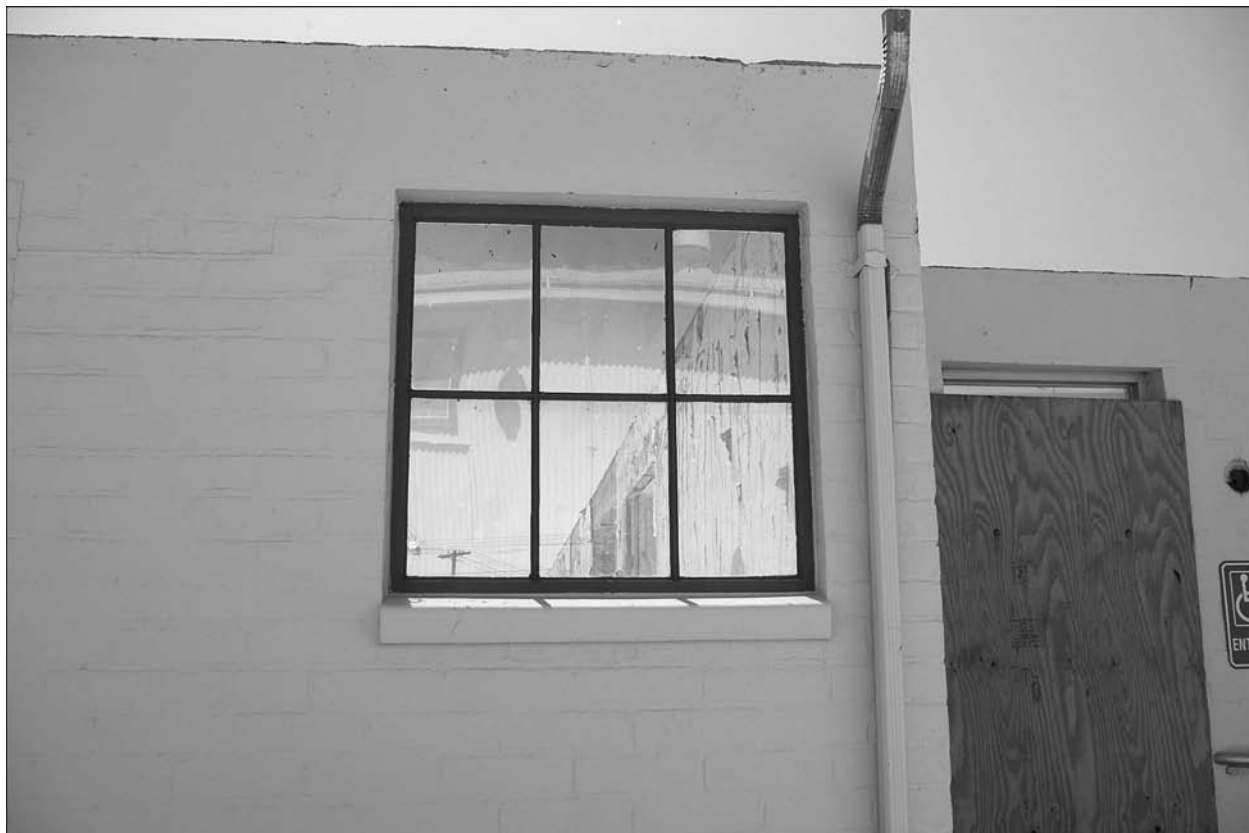
Figure 8. Six-light, steel-sash pivot window (exterior of Window 31), August 2007.
