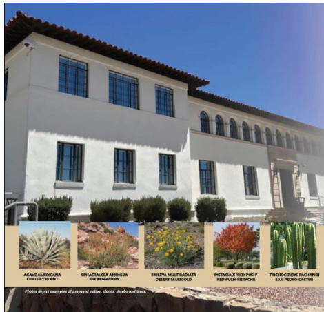
Images of example proposed native plants, shrubs, and trees for the xeriscape project.
