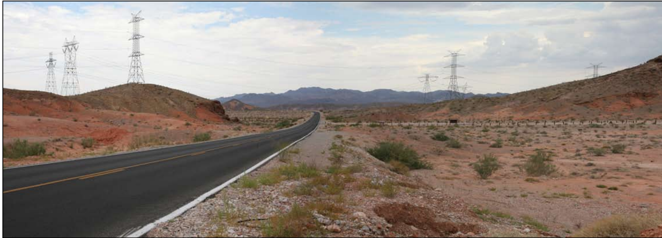
Existing Condition - Existing IPP 500kV lattice structure transmission line, existing Crystal-McCullough 500kV transmission line (within the Sunrise Mountain Instant Study Area (ISA)) and existing Harry Allen to Mead double-circuit, 500kV transmission line
