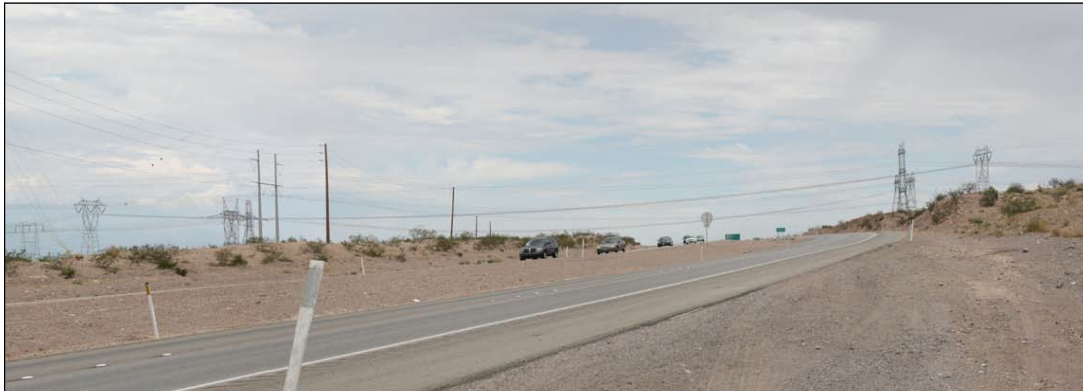
Simulated Condition - Proposed Southern Nevada Intertie Project single-circuit 500kV steel lattice structure transmission line
