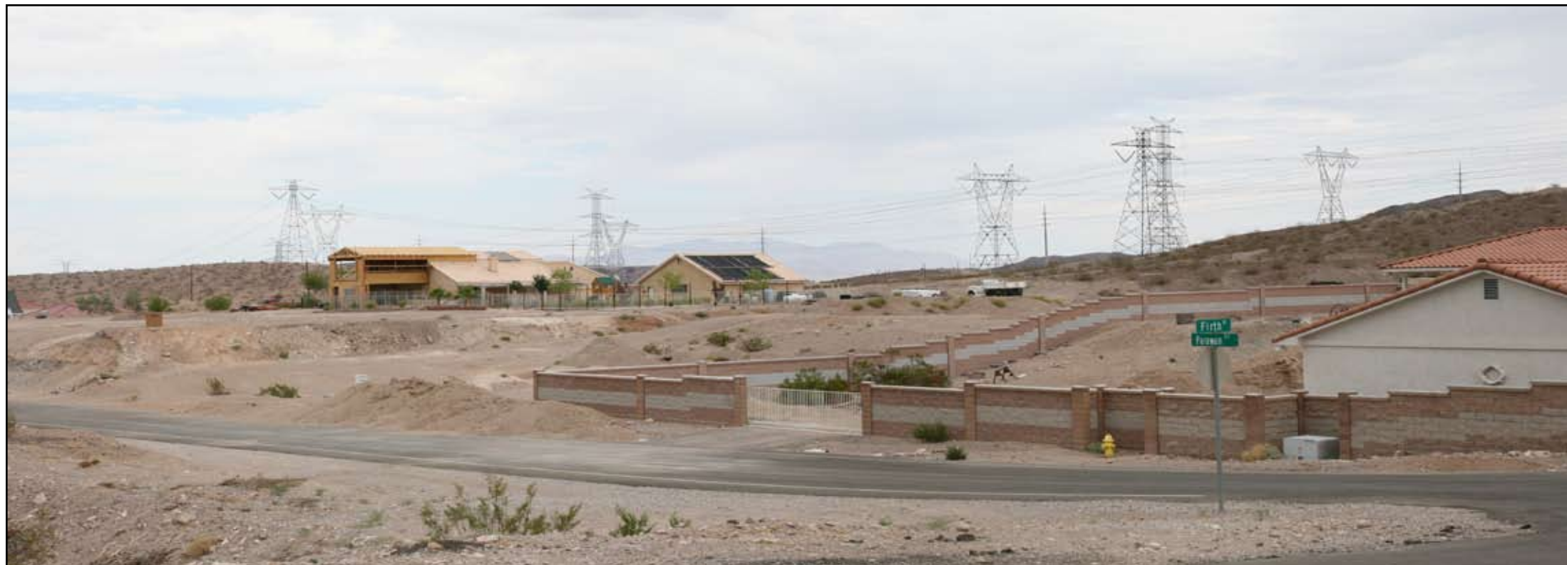
Simulated Condition - Proposed Southern Nevada Intertie Project single-circuit 500kV steel lattice structure transmission line
