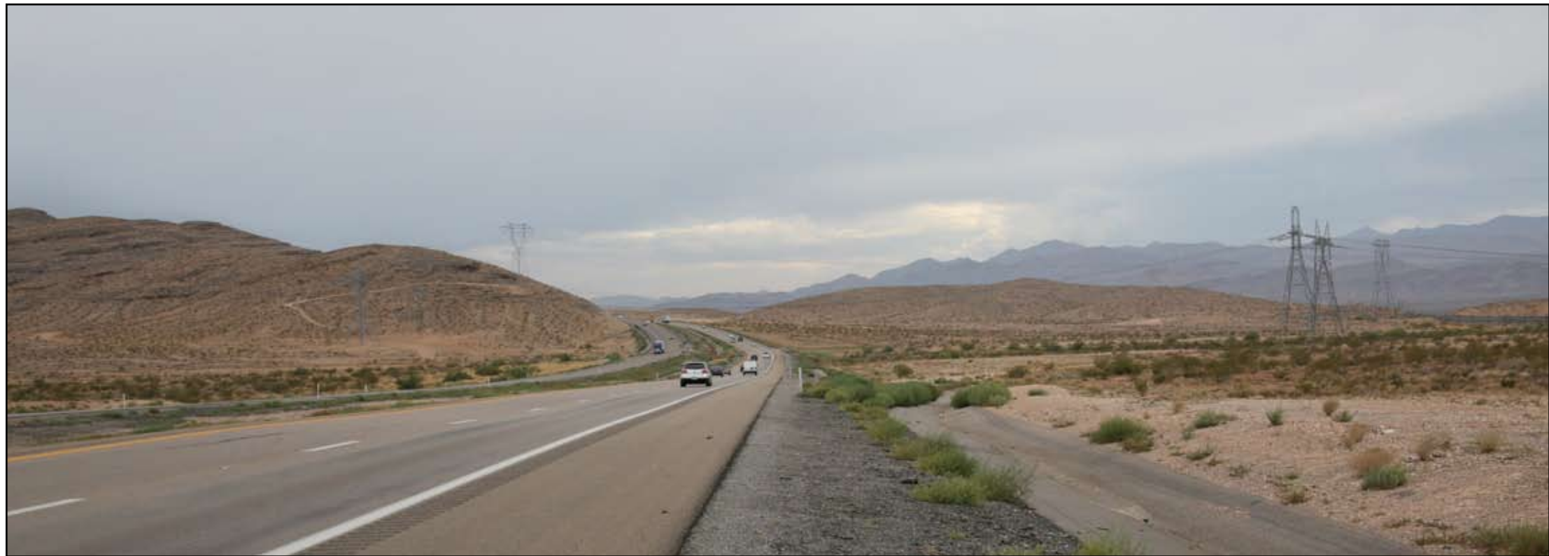
Simulated Condition - Proposed Southern Nevada Intertie Project single-circuit 500kV steel lattice structure transmission line
