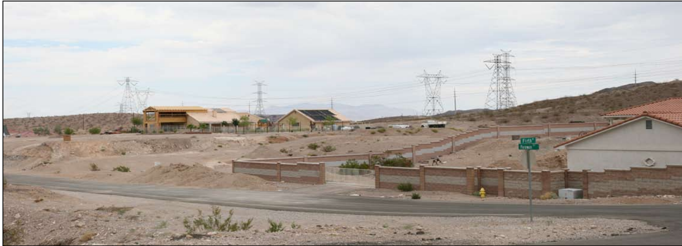
Existing Condition - Existing IPP 500kV lattice structure transmission line, existing Crystal-McCullough 500kV transmission line, existing Harry Allen to Mead double-circuit 500kV transmission line, and existing 138kV line adjacent to Foothills Residential Community
