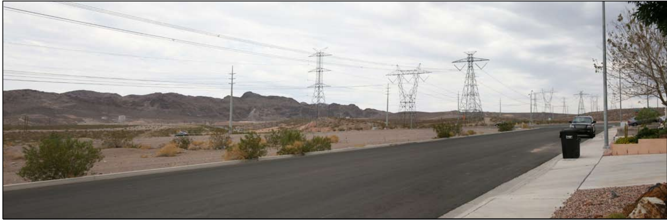
Existing Condition - Existing IPP 500kV lattice structure transmission line, existing Crystal-McCullough 500kV transmission line, existing Harry Allen to Mead double-circuit 500kV transmission line, and existing 138kV line crossing East Lake Mead Parkway and adjacent to the Calico Ridge residential community
