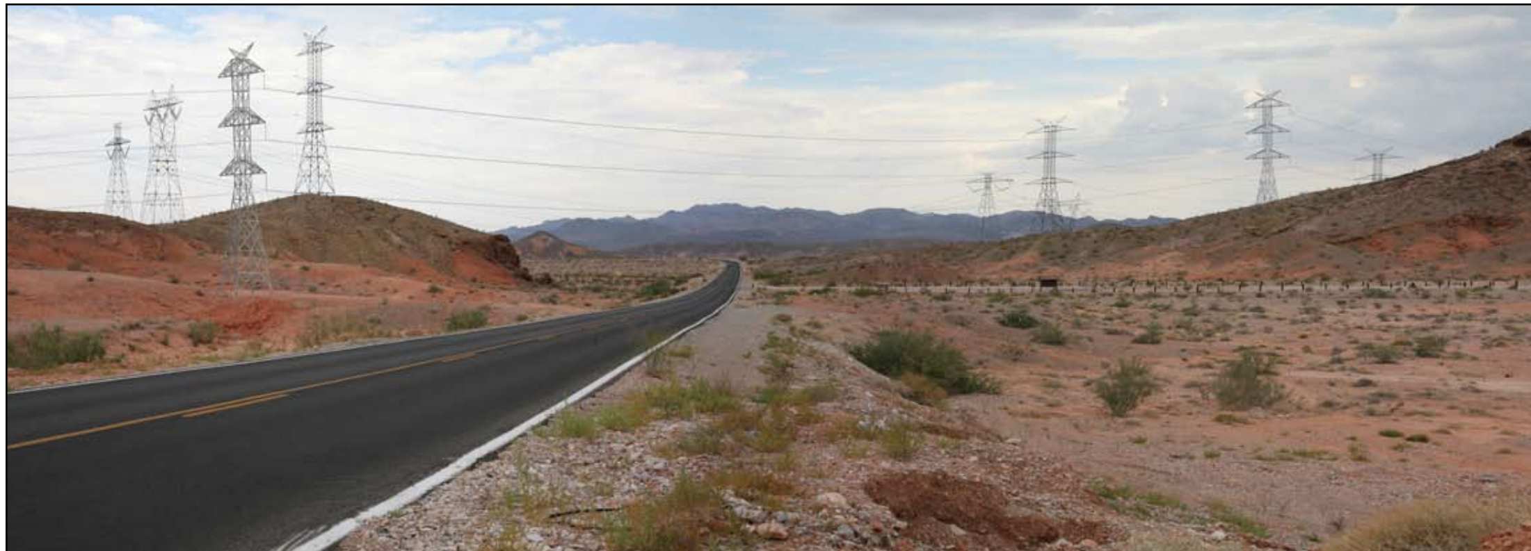
Simulated Condition - Proposed Southern Nevada Intertie Project double-circuit 500kV steel lattice structure transmission line
