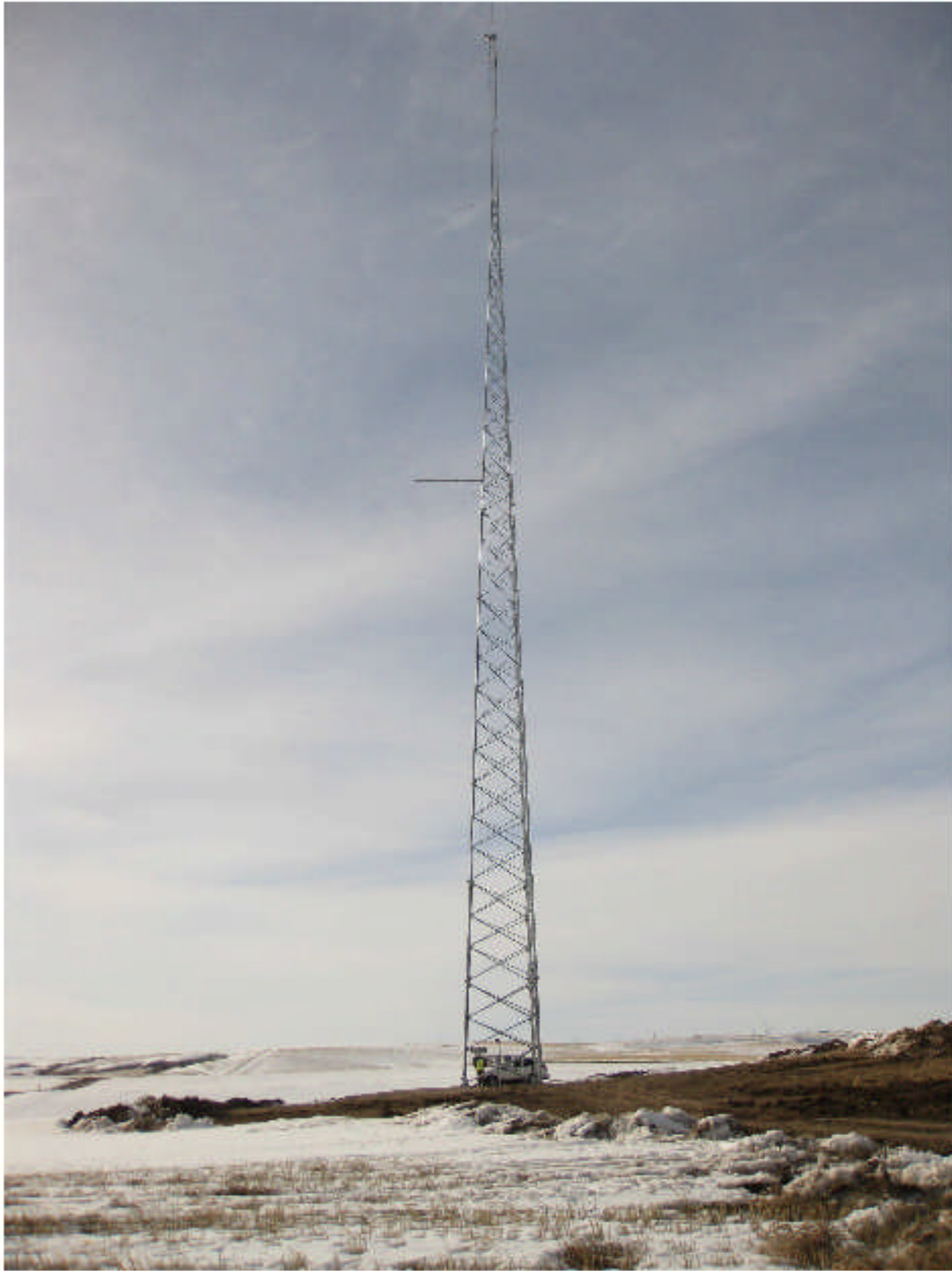
Figure 10. Permanent Met Tower Design (Photo from Idaho Falls, Idaho)
