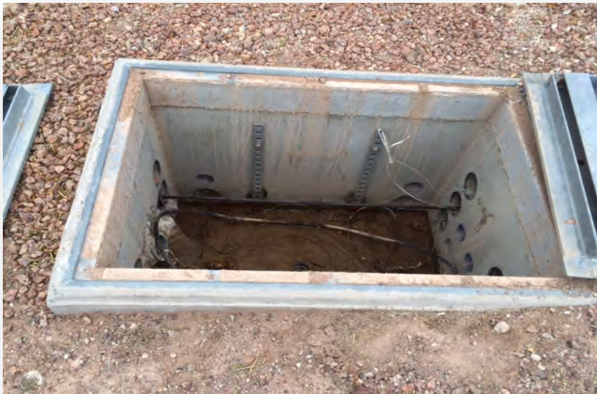
Figure 1- Typical buried Cable vault box
