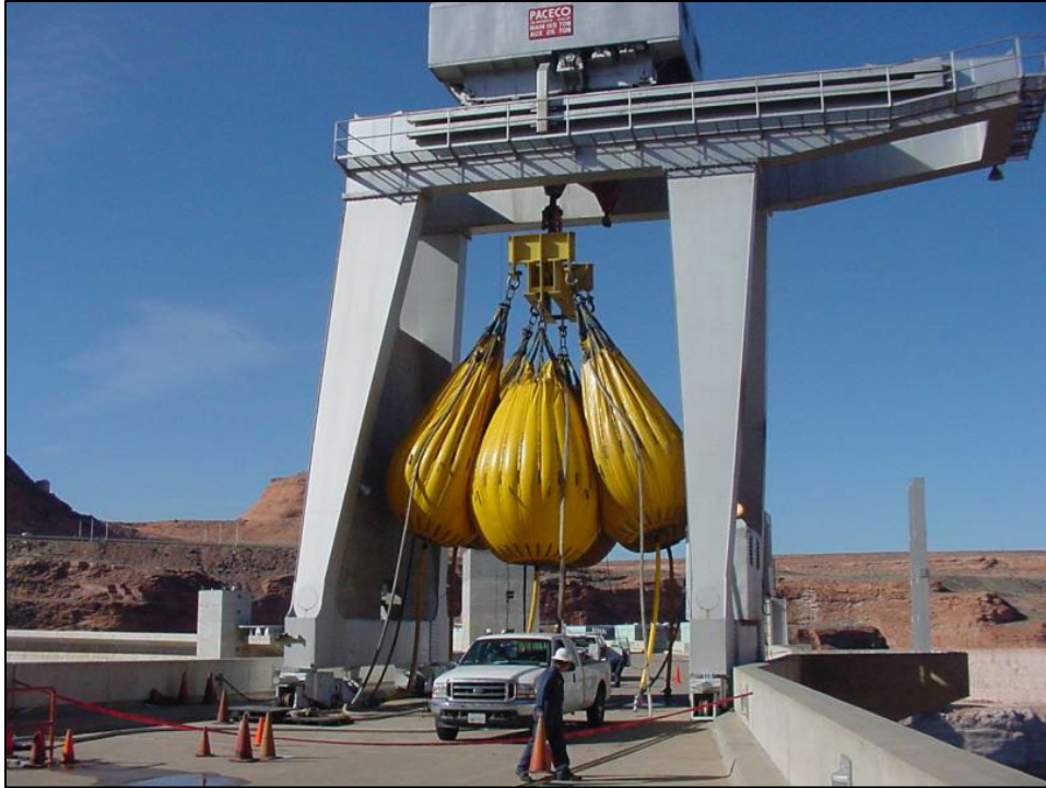
Figure 5. Crane testing at Glen Canyon Dam using water bags (Imes Inc./Gerry Jarin)
