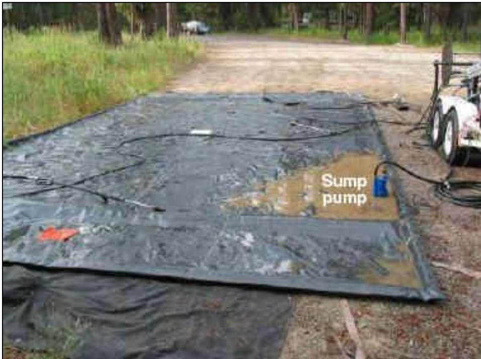
Figure B-1. Bermed portable mat system with sump pump for water recycling (U.S. Department of Agriculture, Forest Service).
