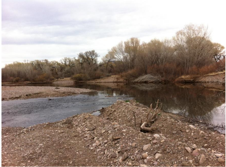
Figure 2-1. Example Push-Up Diversion: Looking Upstream at the Gila Farms Push-up Diversion. The water flowing to the left is directed to the Gila Farms Ditch.
