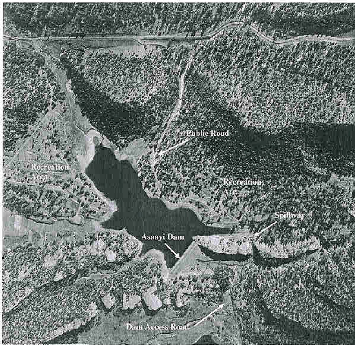
Figure 2. Asaayi Dam and Spillway.
