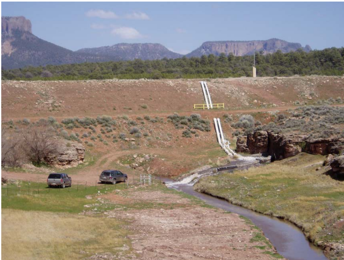
Figure 6. View of siphons on downstream embankment of Tsaile Dam. Siphons were operating at a discharge rate of 20 cfs (April 2005).
