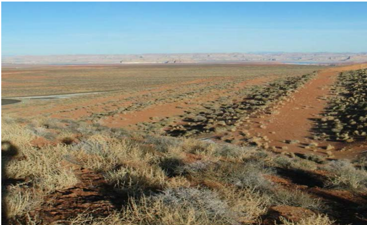
Figure 26 - Terraced Slopes of Ash Disposal Berm.
