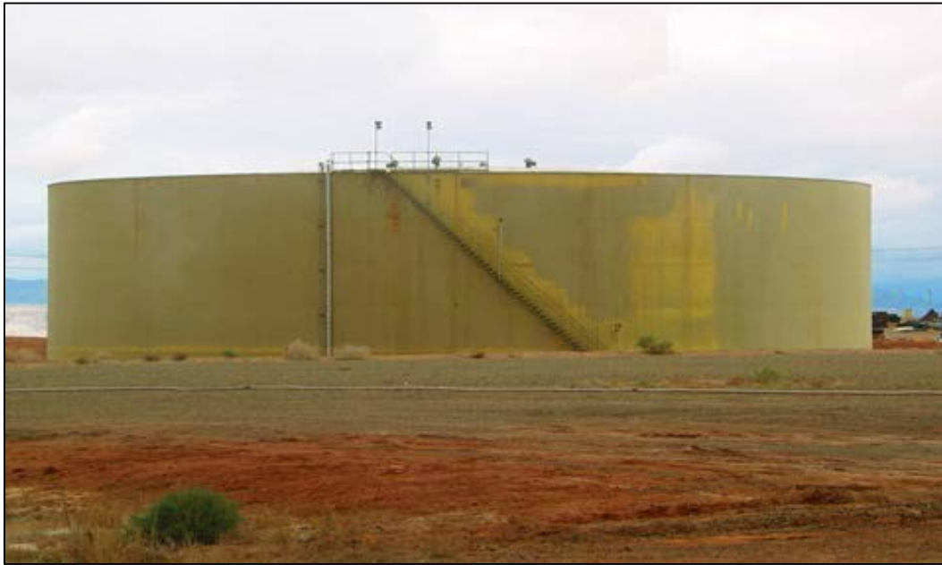
Figure 14 - Primary Fuel Oil Storage Tank.
