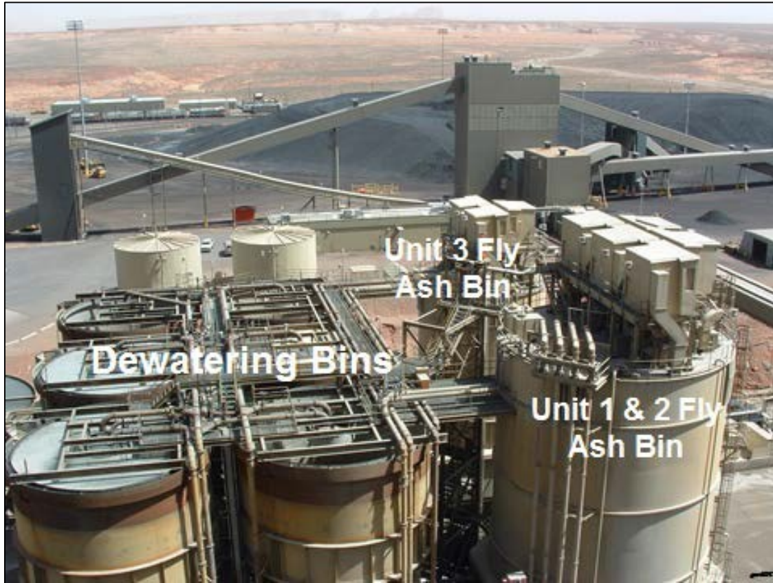
Figure 22 - Ash and Dewatering Bins.
