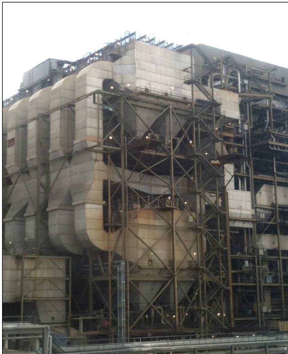
Figure 17 - Hot-side Electrostatic Precipitators (Upper and Lower Decks).
