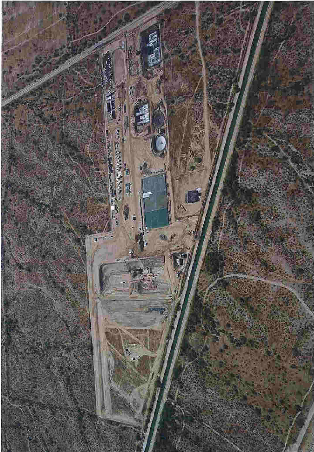
Figure 2-2: Aerial View of the White Tanks WTP While Under Construction (circa early summer 2008)
