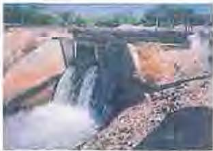
Figure 3-13 Drop at Turnout #9 check structure, Olive Avenue.
