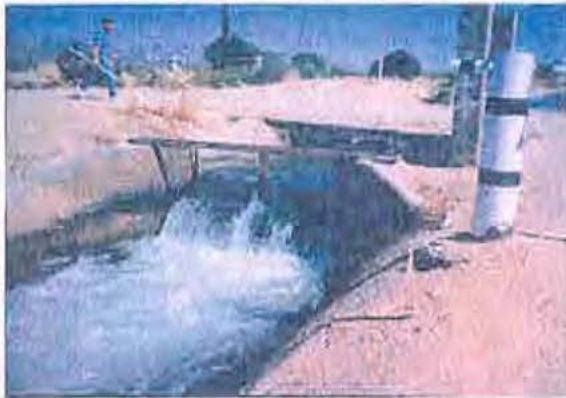
Turnout #10 and CMP culvert under Northern Avenue just upstream of turnout structure
