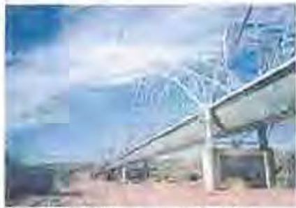
Figure B-9 Flume crossing the Agua Fria River.
