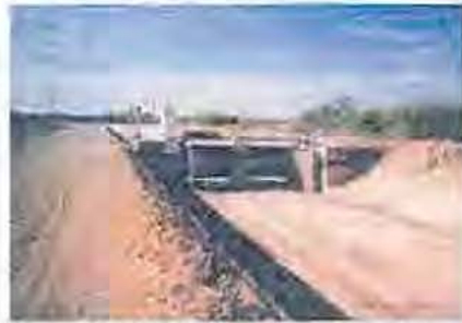
Figure B-11 Radial gate structure upstream of Grand Avenue.
