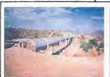
Figure 3-8 Flume crossing of a local wash.
