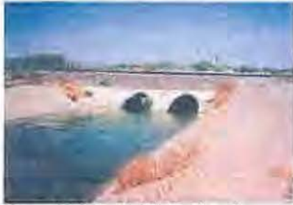
Figure B-6 Santa Fe Railroad crossing - CMP double-barrel culvert.
