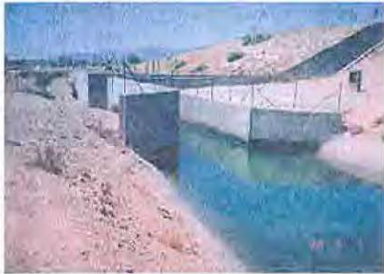
Entrance of inverted siphon at McMicken Dam Chute, McMicken Dam on right.
