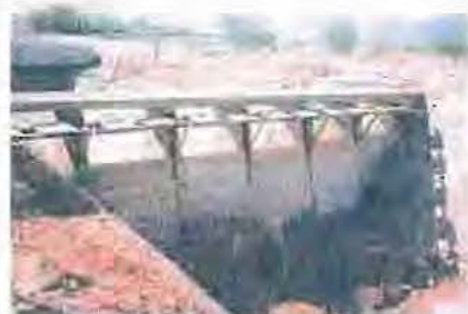
Figure B-13 Checkboard structure for Turnout #4, shown during canal dry-up.
