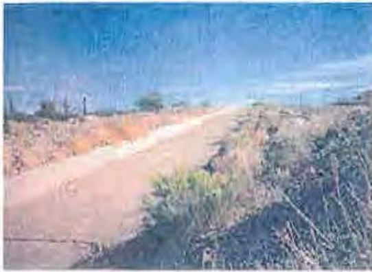
First drop of chute, drops 45 vertical feet. Note canal is 2.5 feet deep.
