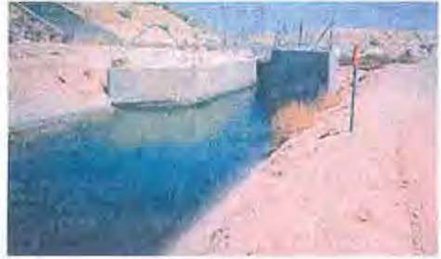
Inverted siphon exit, McMicken Dam on left.
