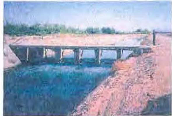
Checkboard structure for Turnout #4, looking upstream.
