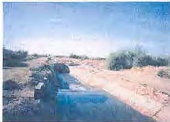
Turnout #12 broadcrested weir, looking downstream and flowing into inverted siphon.
