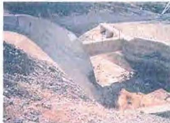
Oblique view of final drop of chute and basin. Start of Agua Fria River Flume at upper right.
