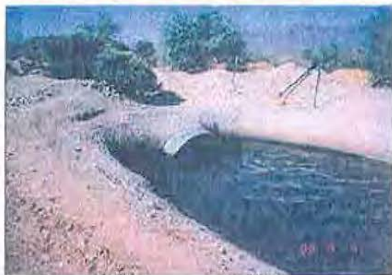
CMP culvert, Turnout #8 checkboard structure inside.
