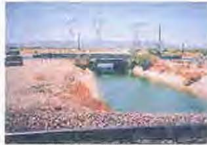
Figure B-7 Grand Avenue crossing - concrete box culvert. Picture taken from Santa Fe Railroad crossing, looking downstream.
