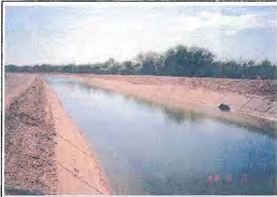
Typical Beardsley Canal cross section above Grand Avenue. Form placed concrete with uniform cross sections. Caved portion at photo right.
