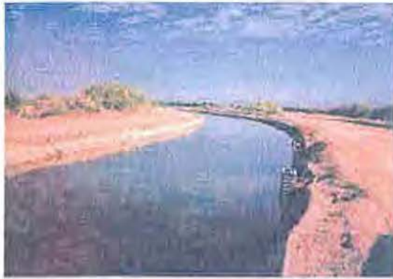
Turnout #5.03, midway between Turnouts #5 and 6
