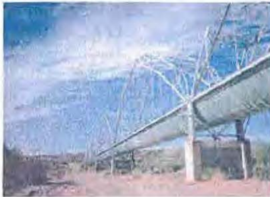
Agua Fria River Flume.
