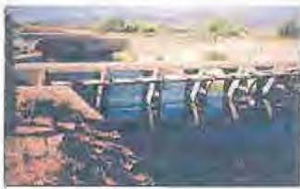
Figure 3-11 Turnout structure for Lateral 4 and the Bell Road bridge.
