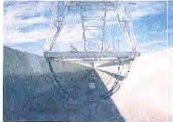
Photograph of inside of Agua Fria River Flume.
