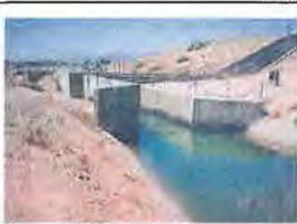
Figure 3-10 Entrance to concrete box inverted siphon under the McMicken Dam chute.
