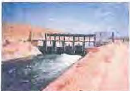
Figure B-12 Sluice Gates for Turnout #3, looking upstream.
