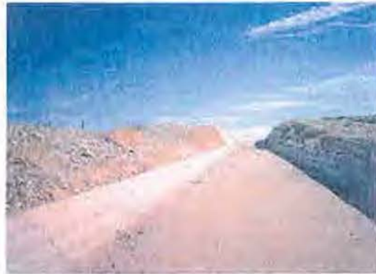
Second drop of chute, drops 33 vertical feet. Note canal is 2.5 feet deep.
