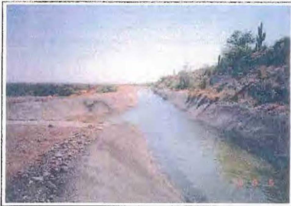
Typical Beardsley Canal cross section above Canal Mile 11. Shotcrete construction, maintenance ramp pictured at left.
