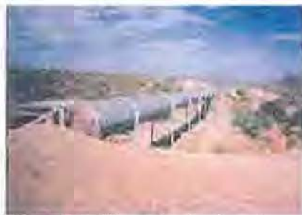
Figure B-8 Flume beginning at station 154080.
