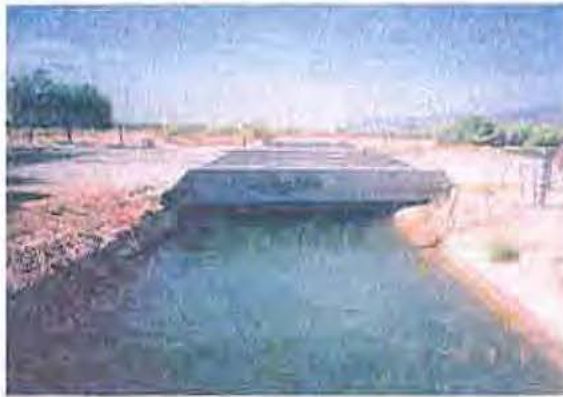
Bell Road Bridge, looking downstream.
