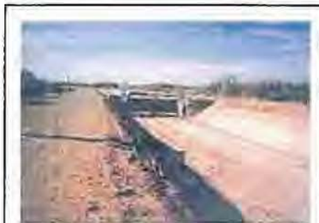
Figure B-2 Example of Beardsley Canal Reach Constructed Using Slip-Formed Concrete. Manning's "n" = 0.015
