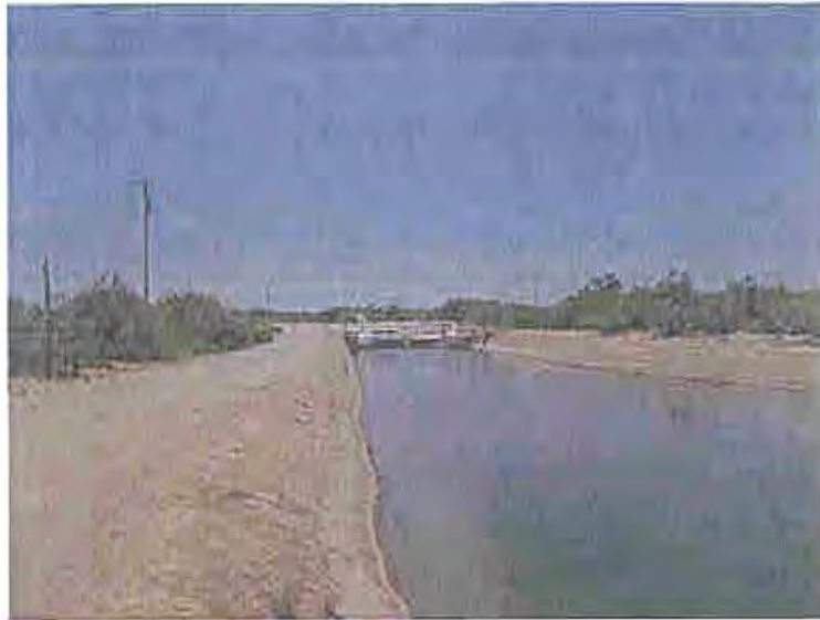
Photo 51 At 14.6 miles, looking at the radial gate.
