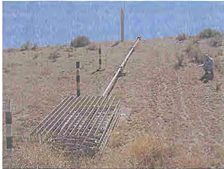
Photo 77 Looking at the sliding gate and shaft in the Trilby Wash Detention Basin.
