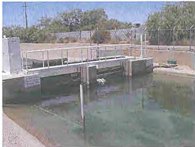
Photo 56 At 17.0 miles, looking at the two radial gates
