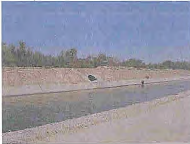
Photo 53 At 15.8 miles, looking northwesterly at the 24 inches CM pipe at the west side of the Canal
