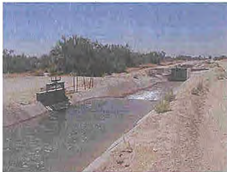
Photo 78 At 30.1 miles, looking southeasterly at the turnout and inverted siphon under the cross drainage channel between Bethany Home Road and Camelback Road
