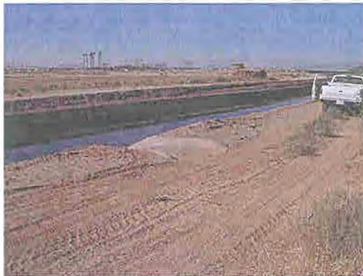
Photo 62 At 18.2 miles, looking southeasterly at the concrete spillway inlet from the road to the Canal. The similar inlet is placed at the 0.1 miles downstream from this point. No photo is taken.
