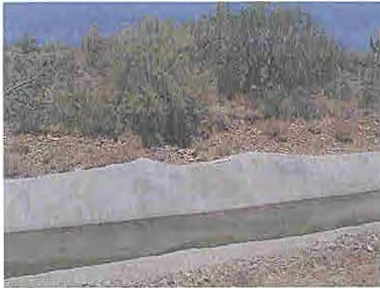
Photo 41 At 7.6 miles, looking westerly at the concrete waterway into the Canal from the hill
