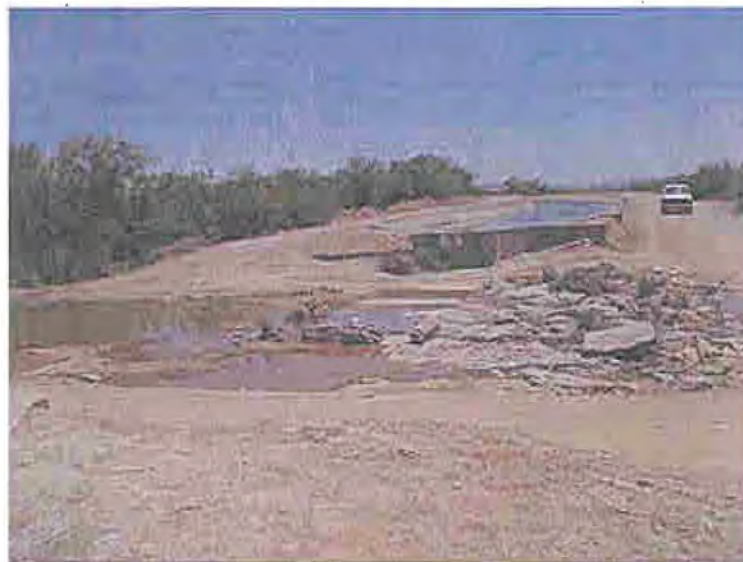
Photo 50 Looking northerly at the headwall of the inverted siphon in the Photo 48.
