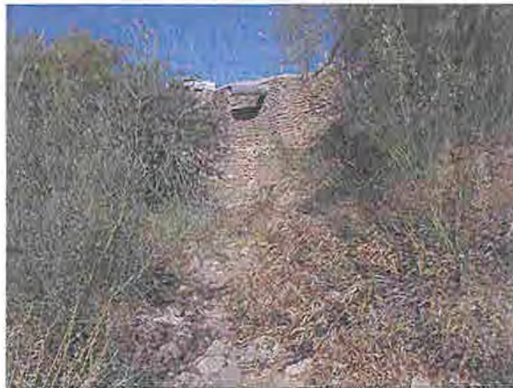
Photo 10 At 1.4 miles, looking from east side of Canal at the 5 feet by 5 feet box culvert inlet under the Canal road. The protruding 12 inches CM pipe is a drain pipe from the 2 feet by 2 feet grate catch basin at the east edge of the road to capture road runoff.
