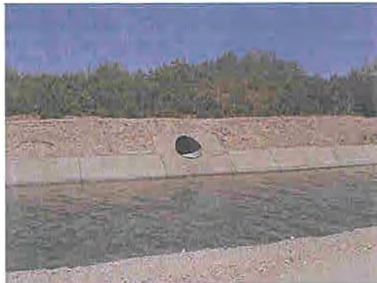
Photo 52 At 15.6 miles, looking northwesterly at 24 inches CM pipe at the west side of the Canal.
