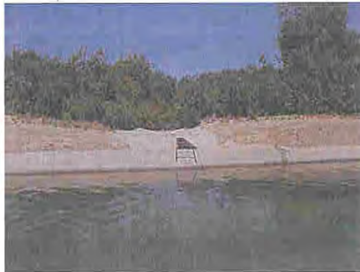
Photo 54 At 16.0 miles, looking westerly at the concrete lined waterway into the Canal at the west side
