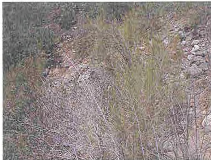
Photo 42 At 8.0 miles, looking southwesterly from east side of the Canal at the 18 inches CM pipe exit under the Canal
