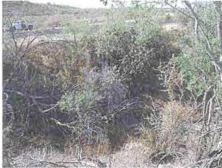
Photo 9 CM pipe exit under the Canal in the middle of the Photo to the Agua Fria River
