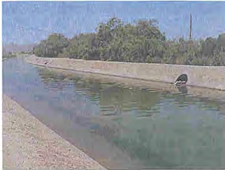
Photo 55 At 16.7 miles, looking southerly at the two beveled 24 inches CM pipes at the west side of the Canal
