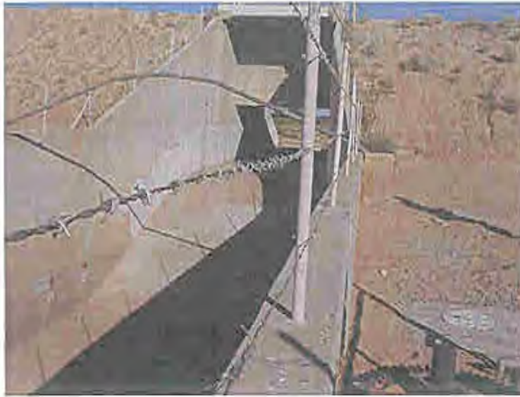
Photo 61 Looking westerly at McMicken Dam Spillway
