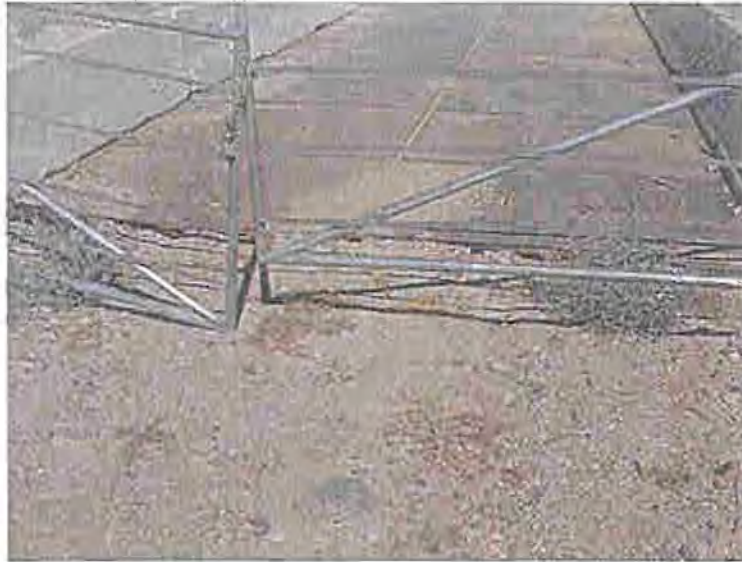
Photo 19 Close look at the steel bridge over Canal
