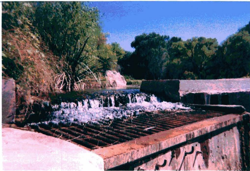
Figure 4. The diversion is located within a two-acre inholding within the Preserve. The grate captures low flows into a pipeline for downstream use by the golf course.
